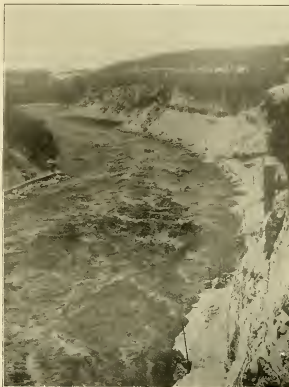
WASHOUTS ON GORGE ROAD.
