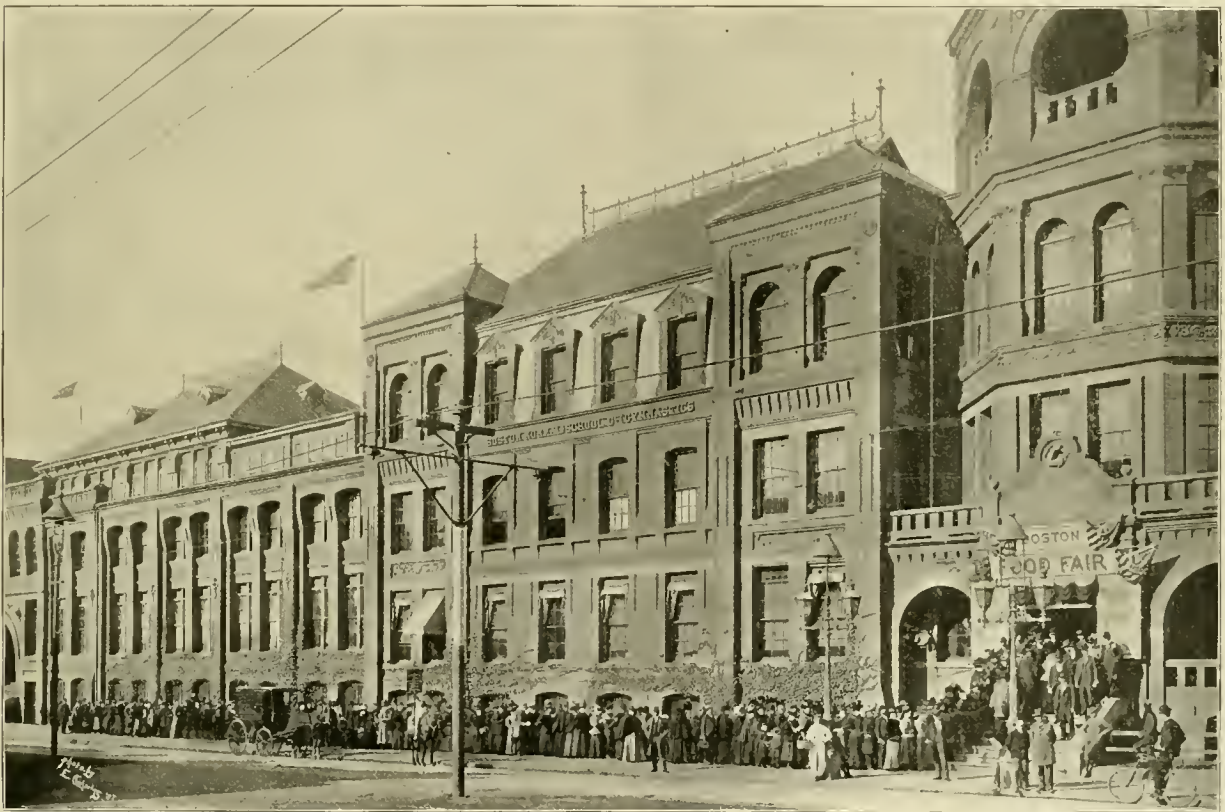
"MECHANICS' BUILDING," BOSTON.
