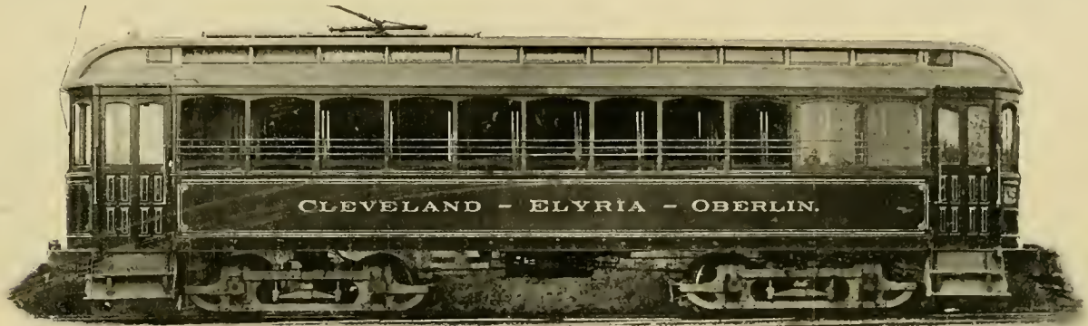
INTERURBAN CAR MOUNTED ON PECKHAM NO. 15 SWIVEL TRUCKS.
