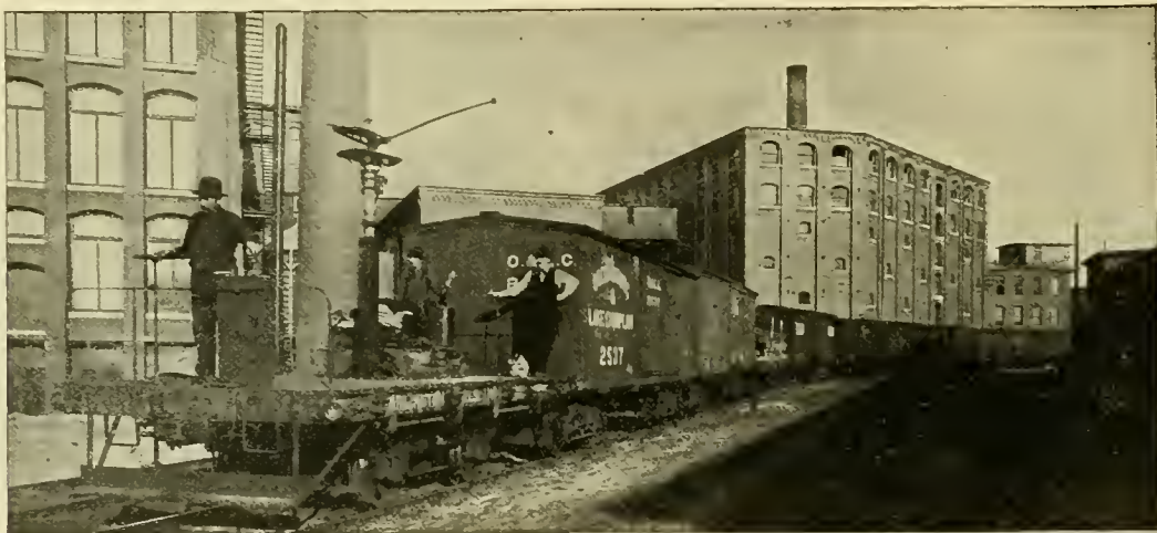
ELECTRIC SWITCHING, ARLINGTON MILLS.
