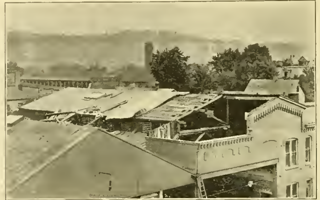
CAR BARN DAMAGED BY WIND STORM.
