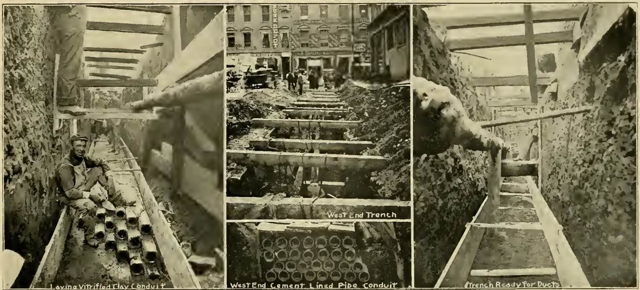
Laying Vitrified Clay Conduit
