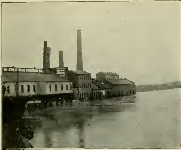
COLUMBUS ELECTRIC LIGHT PLANT.
