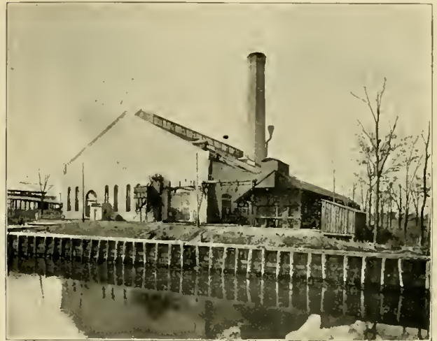
FIG. 2.—COAL HOUSE, CALIFORNIA AVENUE STATION.
