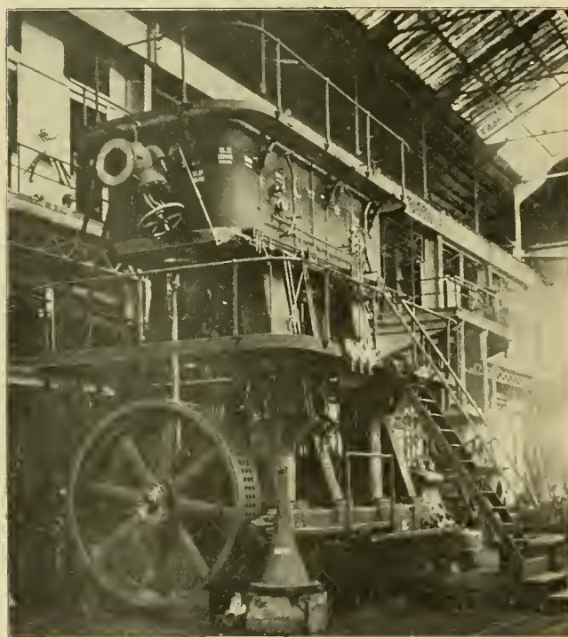
WESTINGHOUSE 2,500-H. P. ENGINE FOR LONDON.
