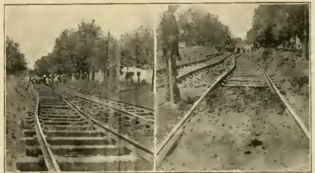
STREET RAILWAY TRACKS BENT BY HEAT.
