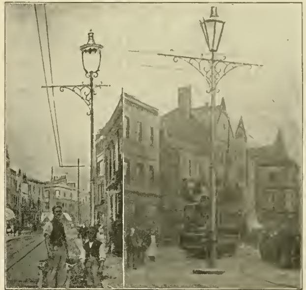
POLES IN DOVER.
