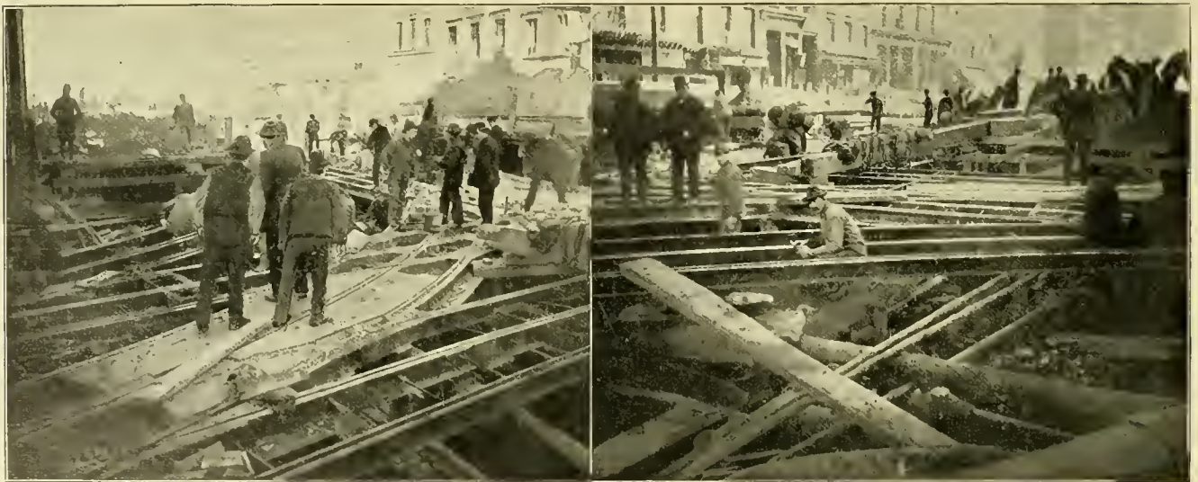
VIEWS OF THE WORK AT WEST BROADWAY AND CANAL STREET.
