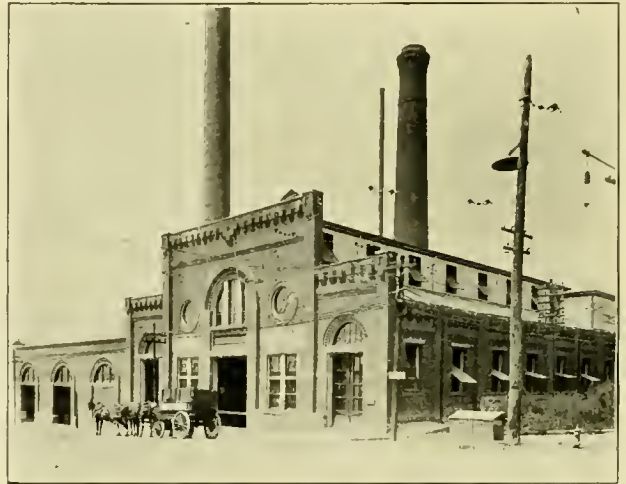
FIG. 1.—HUNT STREET POWER STATION.
