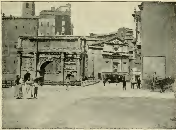
JUNCTION OF VIA BONNELLA AND VIA CAVOUR.
