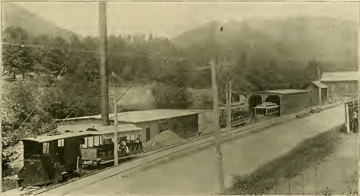
POWER HOUSE AND CAR BARN—SHELBURNE FALLS & COLRAIN STREET RAILWAY.
