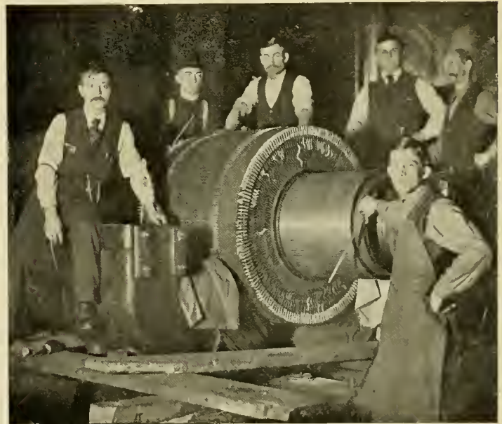
500-K. W. RAILWAY GENERATOR ARMATURE REWOUND.
