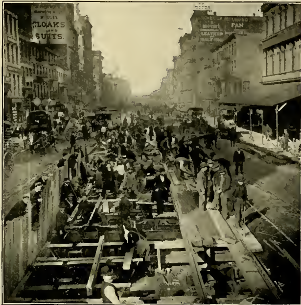
BUILDING THE CONDUIT.
