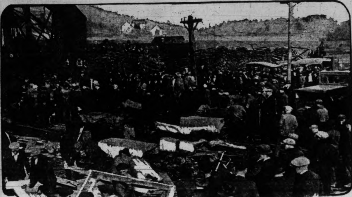
The entrance to the mine near Spangler, Pa., where more than 70 miners were killed by gas explosion and cave-in, was converted into a temporary morgue as victim after victim was brought out of the pit. The linen-covered bodies are shown lying on cots and raised plans waiting for identification and removal for burial.
