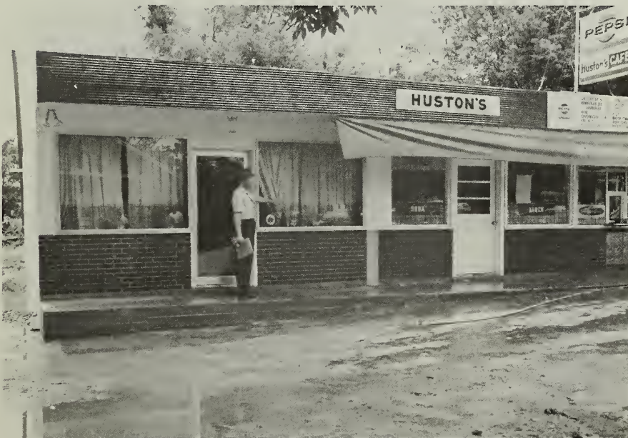
This cafeteria was closed to the public. This is a typical scene in Red Boiling Springs immediately after the rampaging floodwaters swept through town. Loss of business and sanitation problems are economic damages to small businessmen.
