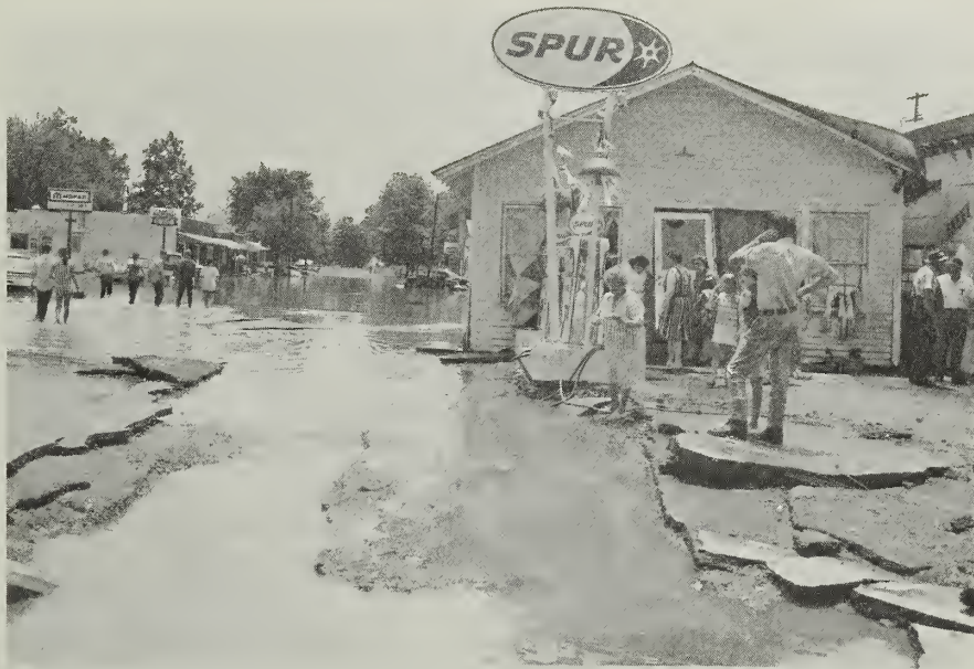
Service station pumps served as brakes for a home washed from its foundation and floated more than a block down the street.
