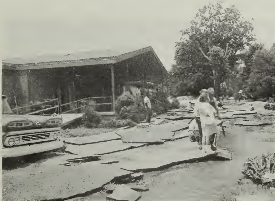
Asphalt pavement from the parking lot and streets was piled five layers deep in front of the Palace Rest Home. Floodwater carried the pickup truck downstream about a half mile where it lodged on the chair ramp of the rest home. Practically all of the lawn and shrubbery was destroyed as floodwater entered the Palace.
