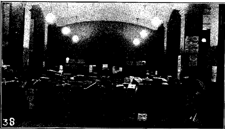
Fig. 18.—Parcel post racks in the General Post Office illuminated by unit No. 4 with a 300-watt lamp, the illumination on the working plane being 8.2 foot-candles
