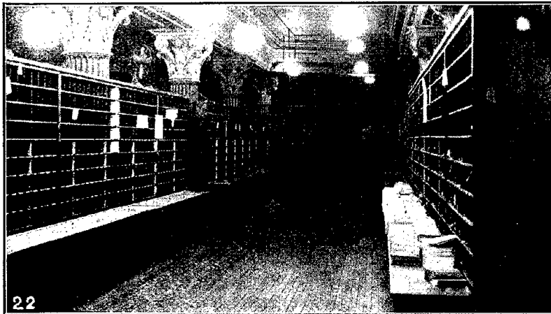
Fig. 15.—Letter separation cases illuminated by unit No. 2 with a 200-watt lamp, the illumination on the horizontal working plane being 6.5 foot-candles
