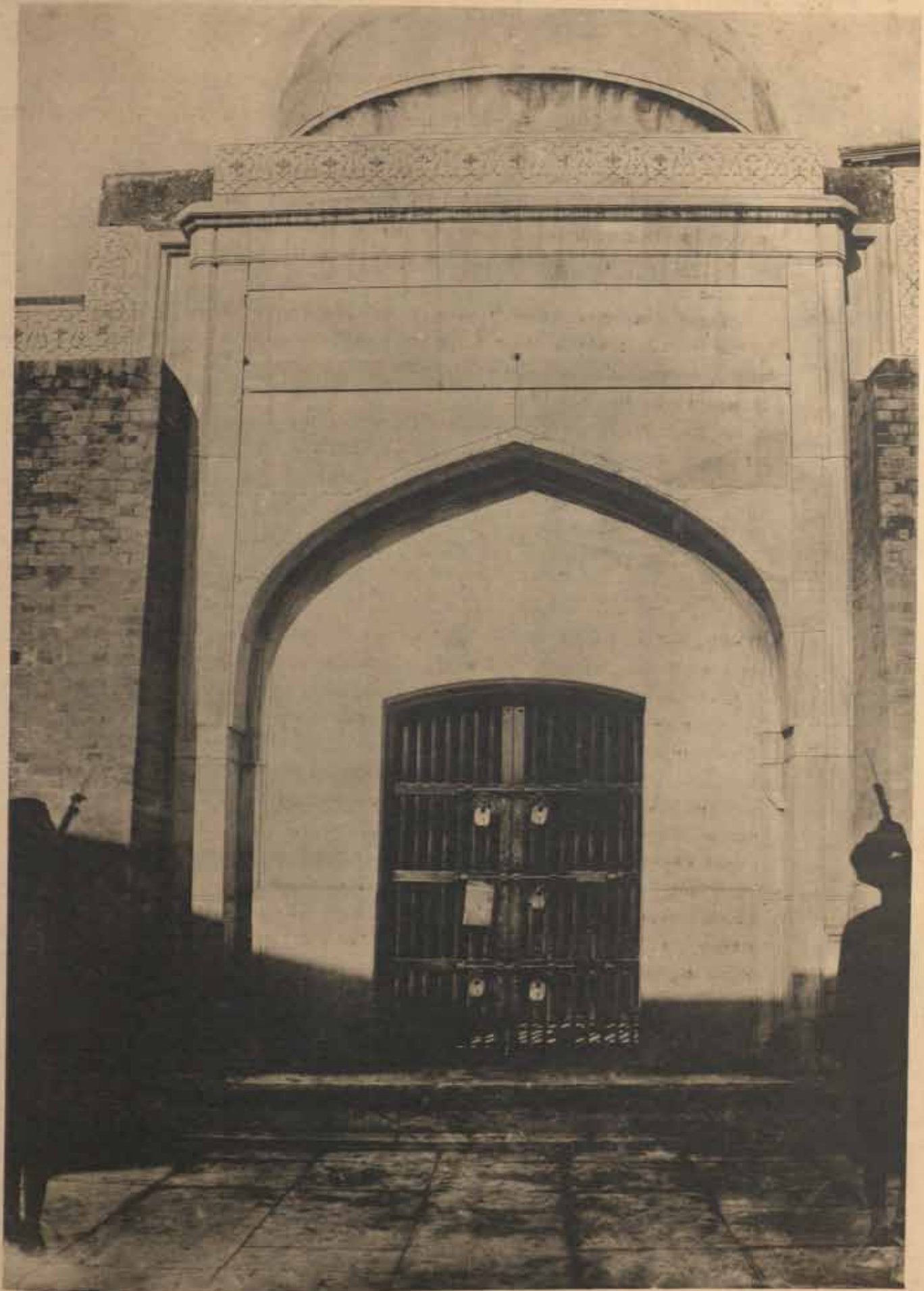
CENTRAL ENTRANCE, BEFORE RESTORATION.
