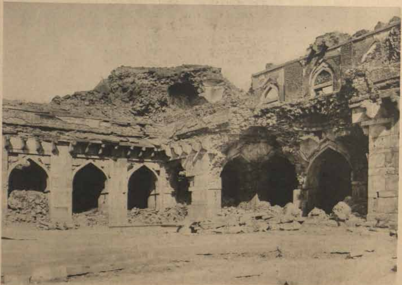
(a) GENERAL VIEW OF BUILDING FROM S.E.
