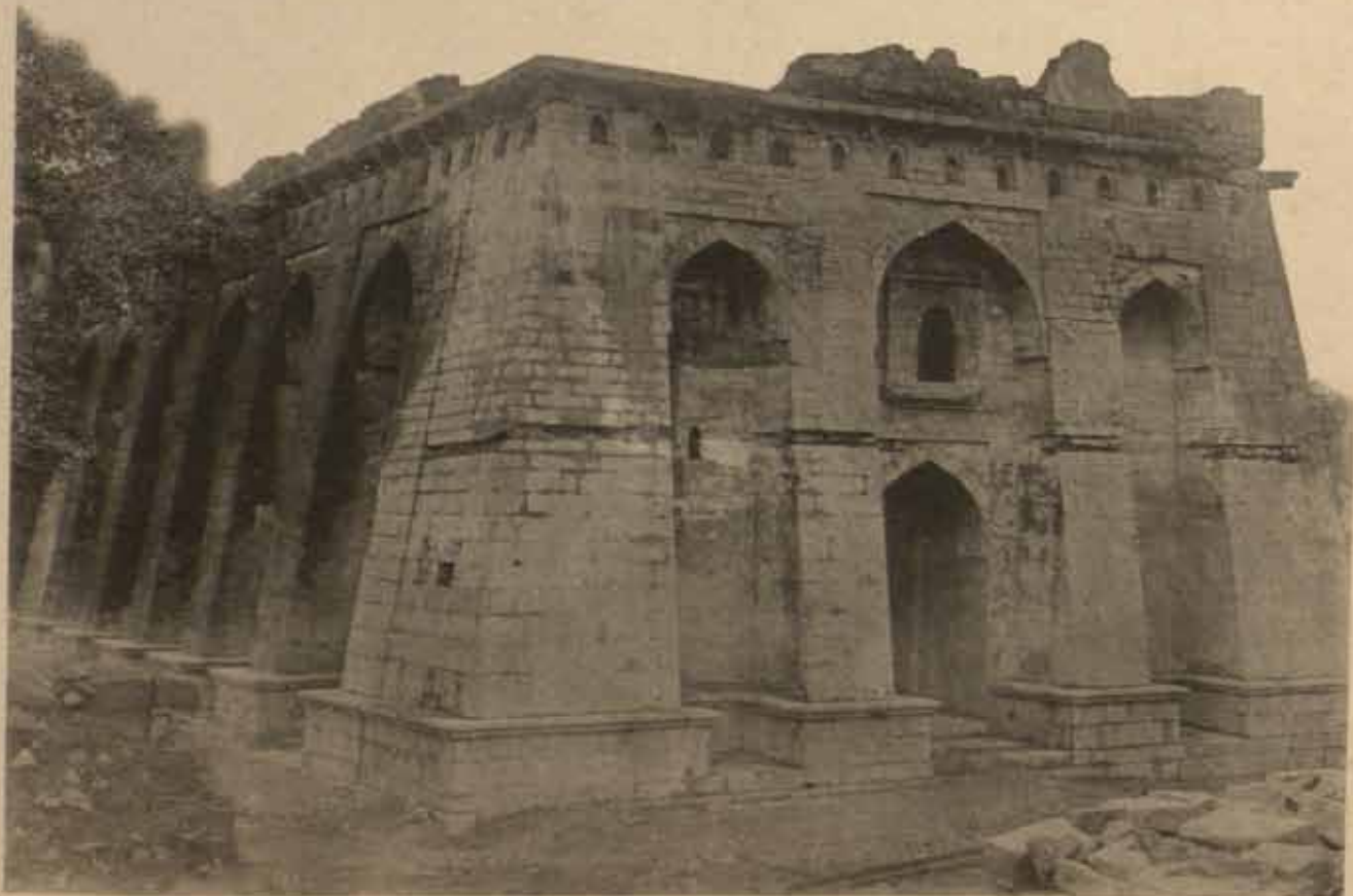
(a) SOUTH END, AFTER DEMOLITION OF LATER STRUCTURE.
