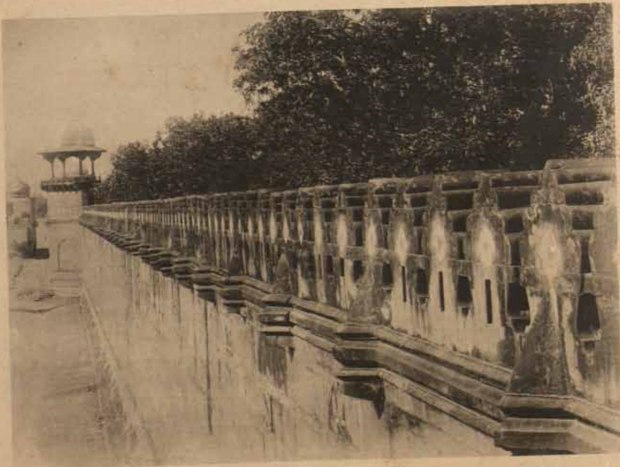
(a) A PANEL IN THE DADO OF THE JAWĀB AFTER RESTORATION. (b) BATTLEMENTS OF THE GARDEN WALL AFTER RESTORATION.
