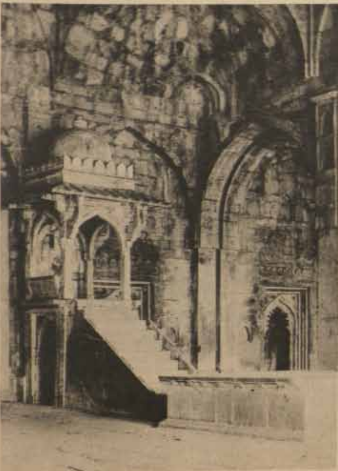
(a) CRUMBLING MASONRY IN THE SOUTH DALĀN, BEFORE REPAIR.
