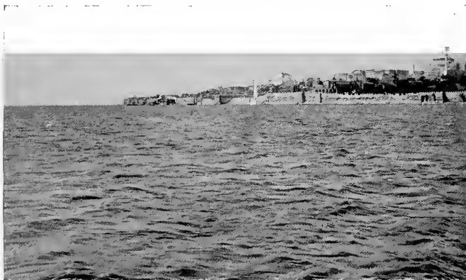
THE SOUTHEAST SEA WALL
