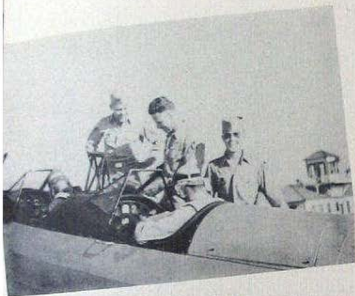
Safety belt fastened?
