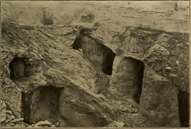
FIG. 1.—View of open cut in magnetite deposit, Mineville, N.Y. The pillars are ore left to support the gneiss hanging wall. After Witherbee, Iron Age, Dec. 17, 1903.
