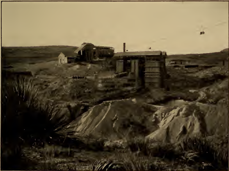
FIG. 2. — Furnace for roasting mercury ore, Terlingua, Tex. W. H. Turner, photo.
