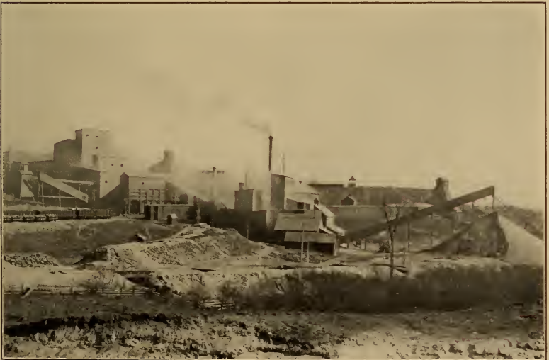
FIG. 2.—General view of magnetic separating plants and shaft houses, Mineville, N.Y. After Witherbee, Iron Age, Dec. 17, 1903.
