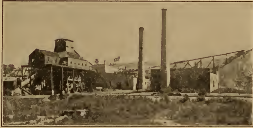
FIG. 10. — Shaft house and tipple, bituminous coal mine, Spring Valley, Ill.
