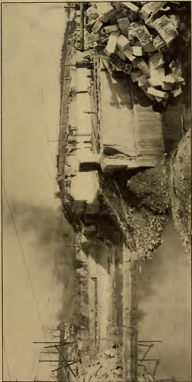
Quarry in limestone, Bedford, Ind. Photo., Bedford Quarries Co. A horizontally bedded limestone, showing some weathering along the vertical joint planes.
