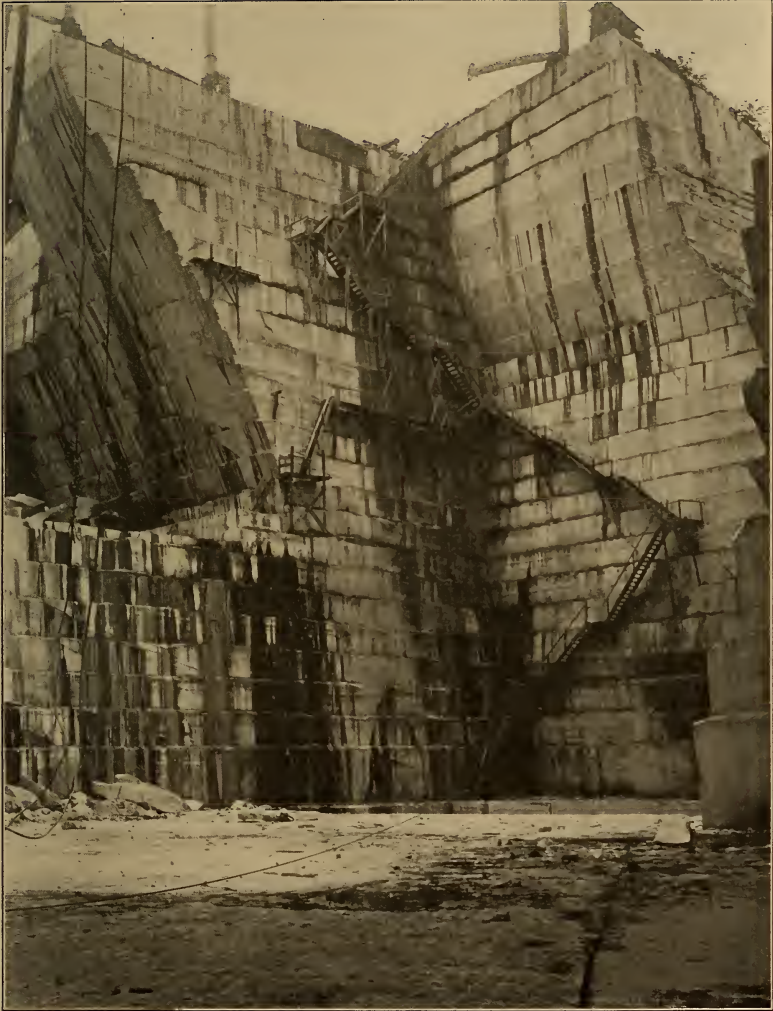
Marble quarry, Proctor, Vt. Photo., Vermont Marble Co. The banding of the rock is vertical. The horizontal lines are caused by the stone being quarried in benches.
