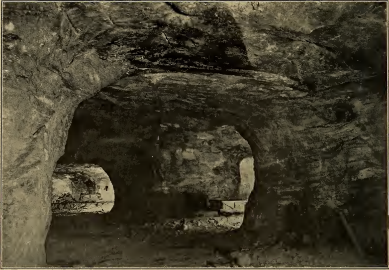
FIG. 1. — Interior view of salt mine, Livonia, N.Y. Both roof and pillars are rock salt.
