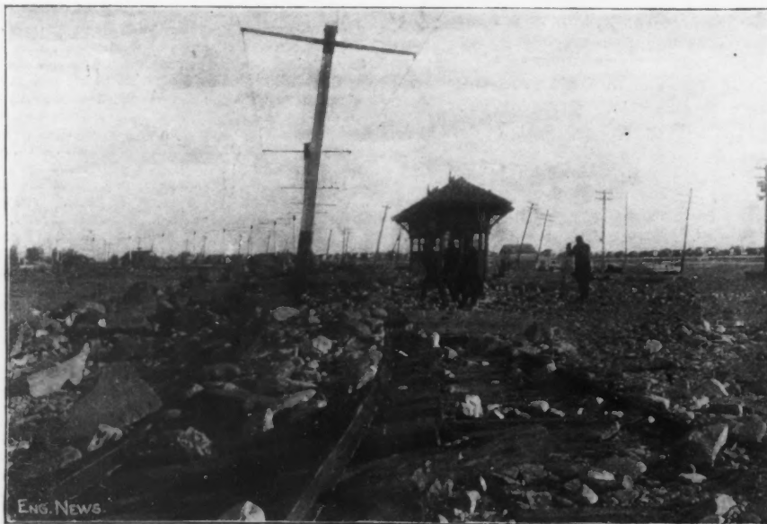
FIG. 1.—VIEW SHOWING SECTION OF RAILWAY TRACK DISPLACED BY OCEAN WAVES; NEW YORK, NEW HAVEN & HARTFORD R. R.
