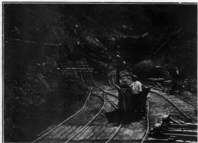
BOTTOM OF INCLINE AND MOUTH OF TUNNEL AT LOWER LEVEL OF ORISKANY MINE
