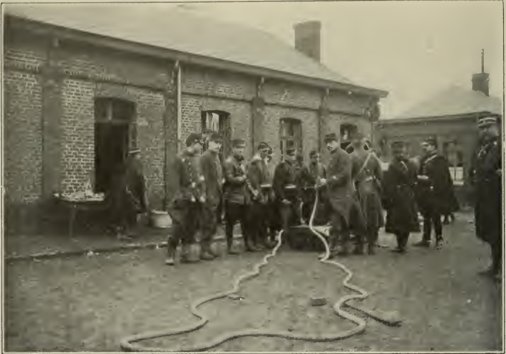
CENTRAL RESCUE STATION ORGANIZED AT THE COURRIÈRES MINES, MAR. 10, 1906.
