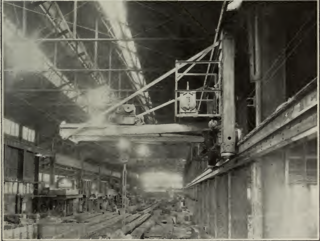
EXAMPLES OF MODERN AMERICAN TRAVELING CRANES.
