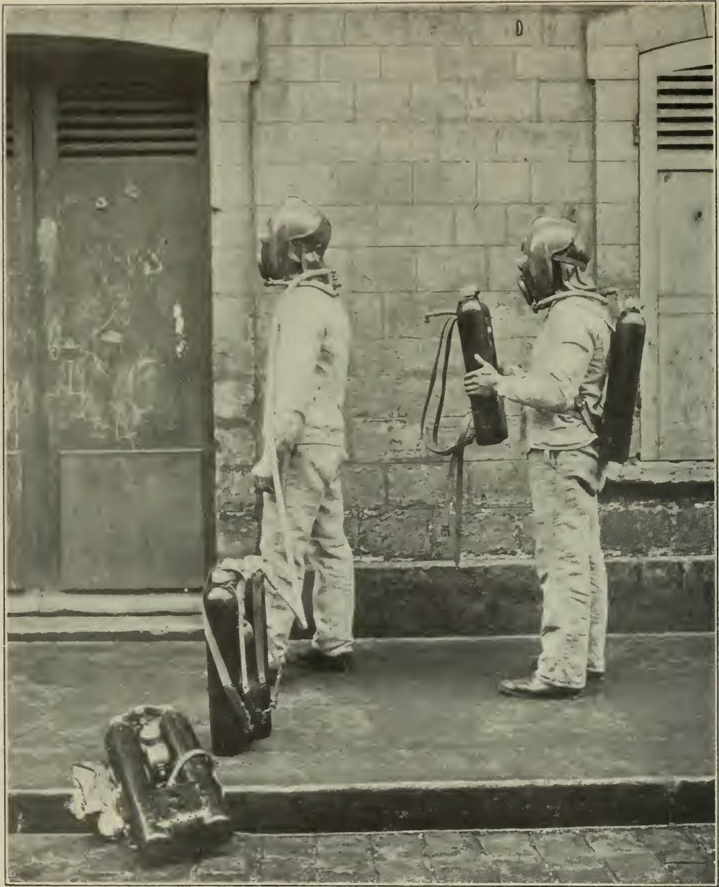
FIG. 13. RENEWAL OF AIR-ACCUMULATOR BATTERIES IN THE VANGINOT APPARATUS.
