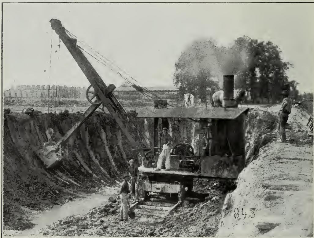
REVOLVING STEAM SHOVEL IN OPERATION.
