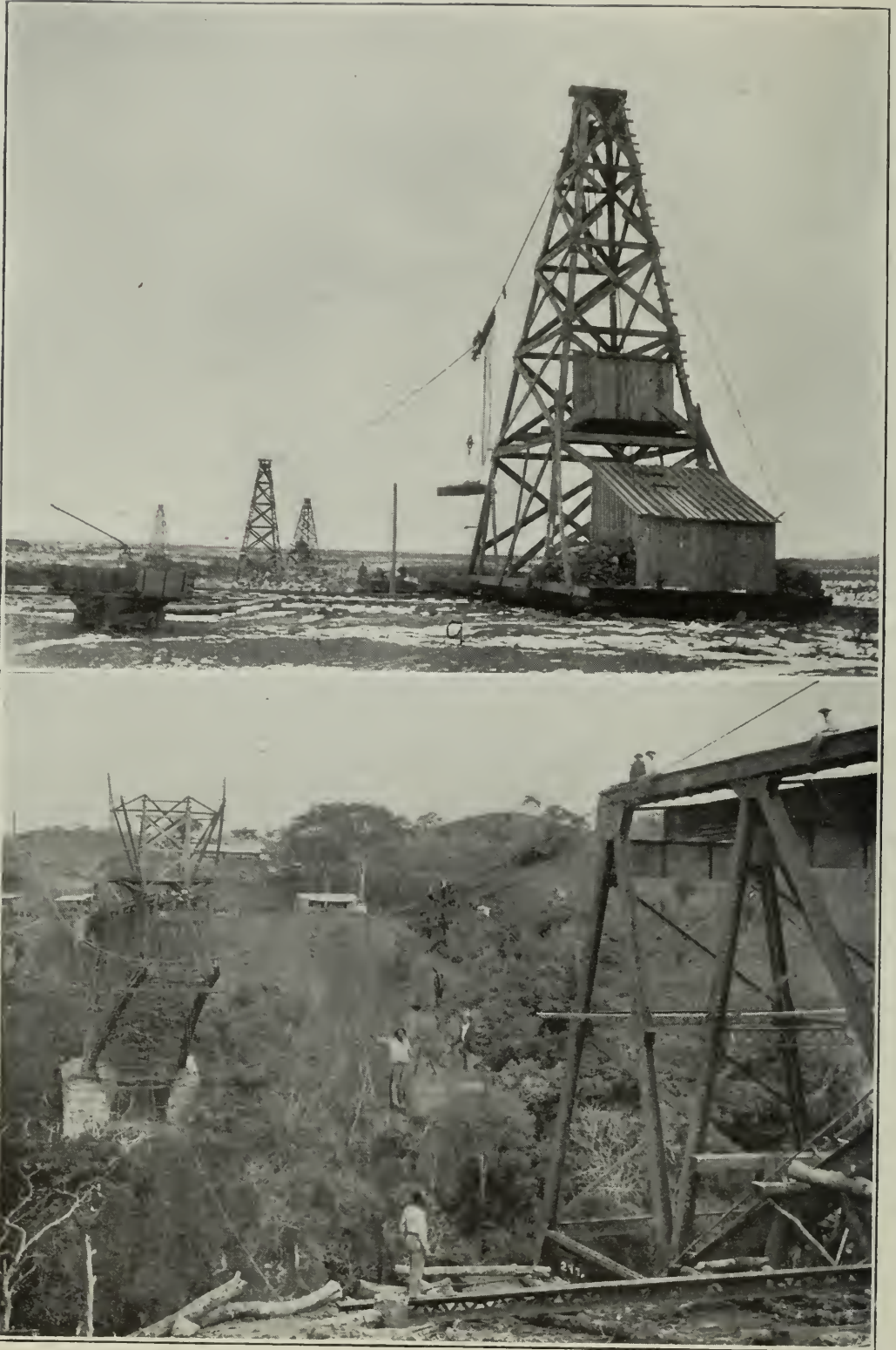
CABLEWAYS IN SERVICE ON CONSTRUCTION WORK.
