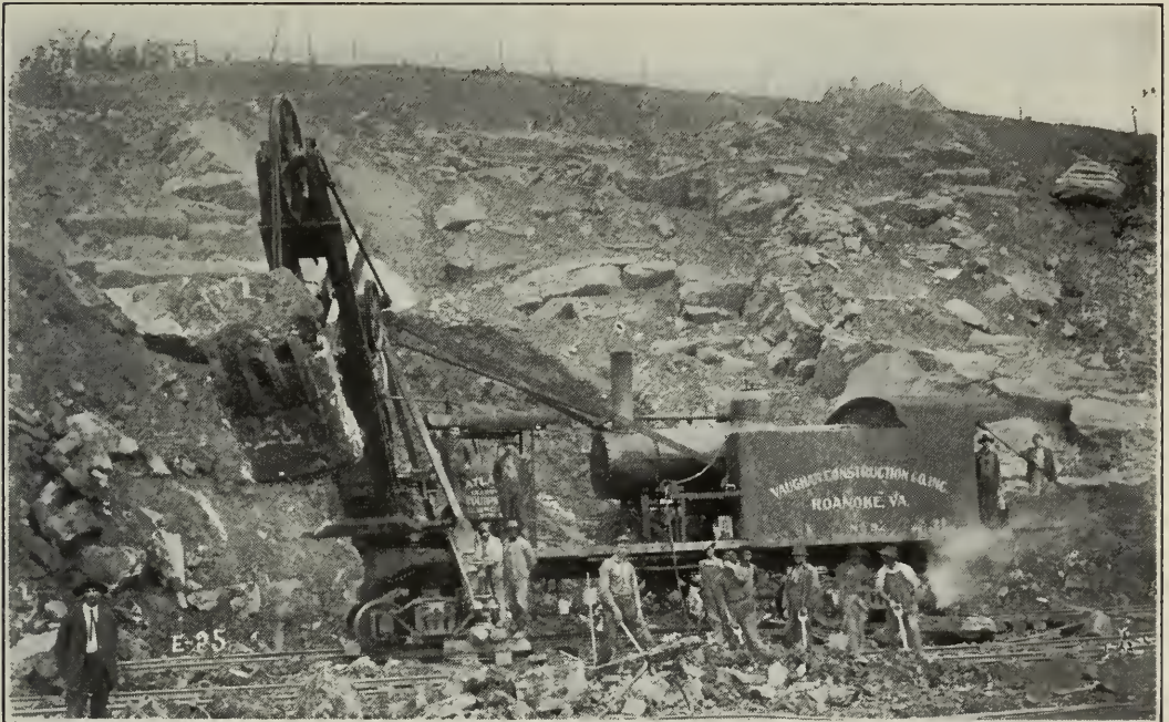
ATLANTIC STEAM SHOVEL AT WORK IN BLASTED ROCK, N. & W. RY. NEAR ROANOKE.
