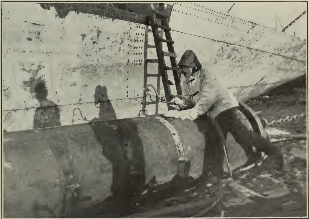
CUTTING A SHAFT BEARING LENGTHWISE.
