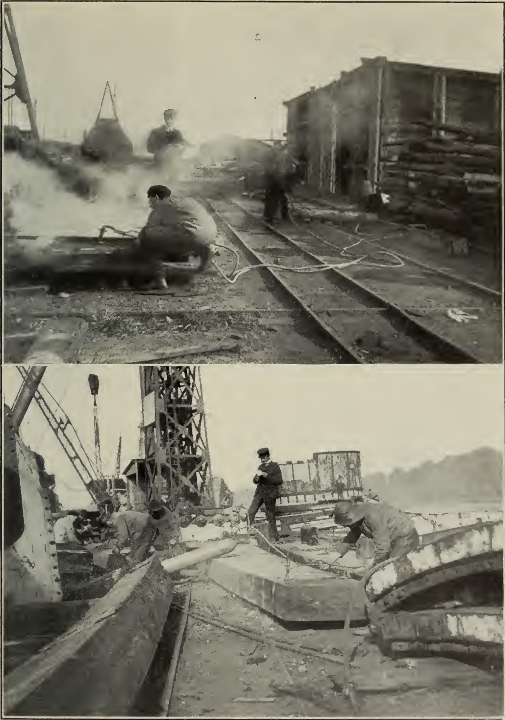
ABOVE, STRAIGHT-LINE CUTTING OF 50-MILLIMETRE PLATES. BELOW, SLOTTING ARMOR PLATE TO A DEPTH OF 6 OR 7 CENTIMETRES.
