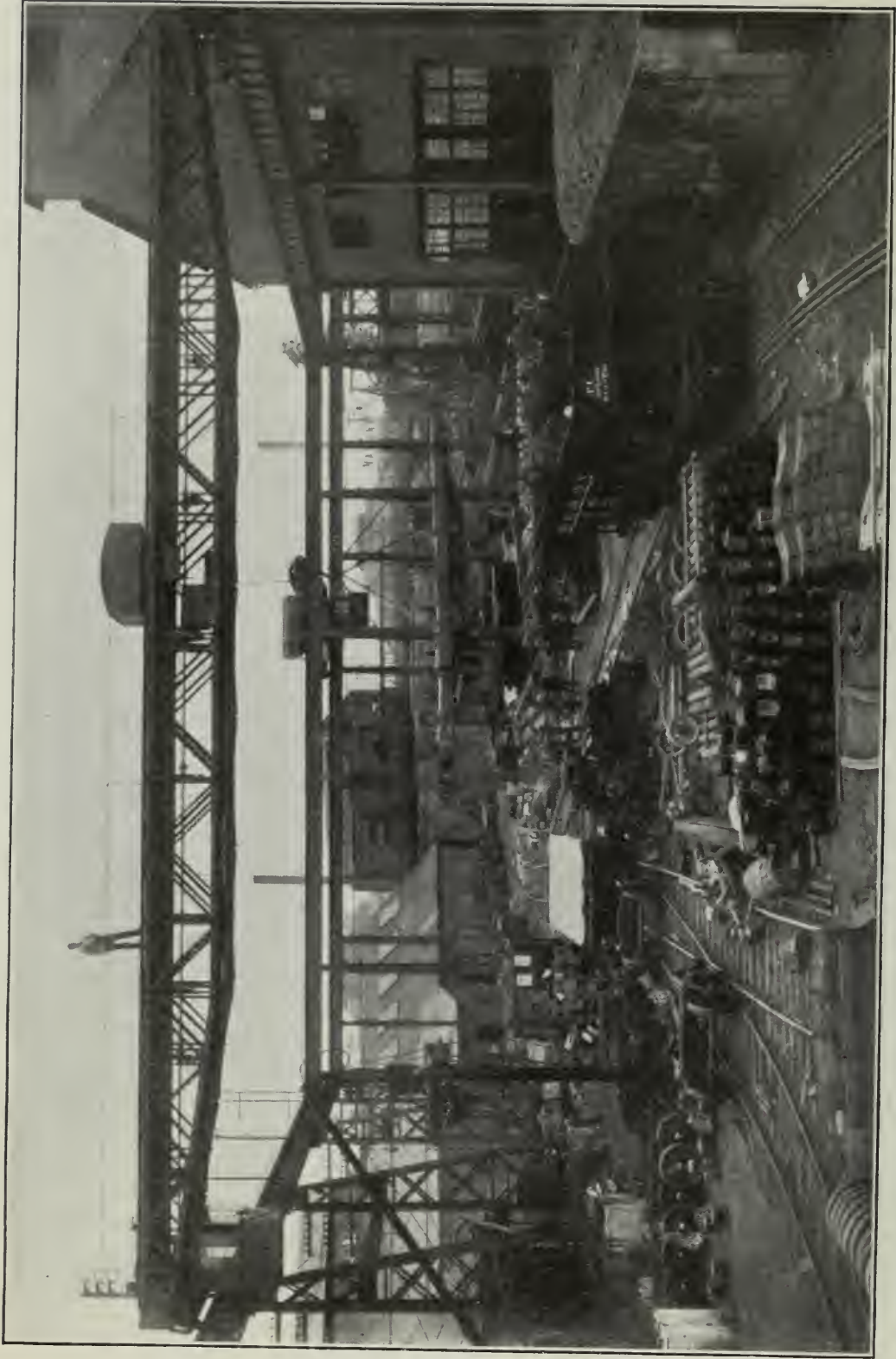
ALTERNATING-CURRENT CRANE, 15-TONS CAPACITY, FOR OUTDOOR SERVICE At the Middletown Car Company's plant. Span 105 ft.; runs on steel elevated runways supported on A-frame posts; latticed bridge-girder construction was adopted to reduce wind pressure and keep down weight. "Northern" type trolley, covered; operators' cab enclosed. Northern Engineering Works.
