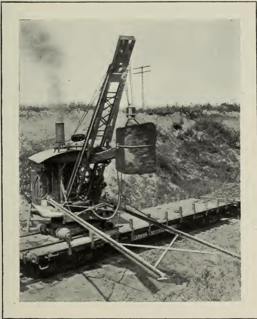
DITCHER, BUILT TO OPERATE FROM A FLAT CAR OR FROM THE GROUND.
