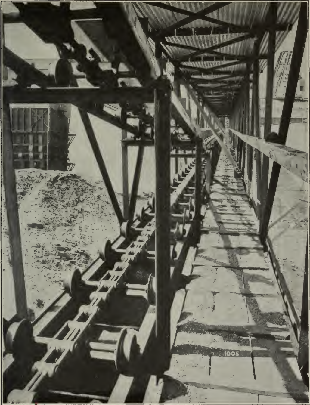
ROLLER CHAIN CONVEYORS FOR CARRYING COAL, CAMDEN COKE CO.
