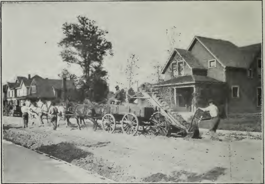
PORTABLE LOADER AT WORK ON STREET GRADING.
