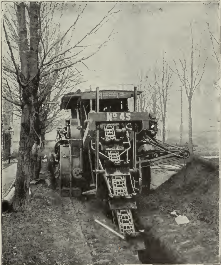
A DITCHING EXCAVATOR IN OPERATION, The Municipal Engineering & Contracting Co.
