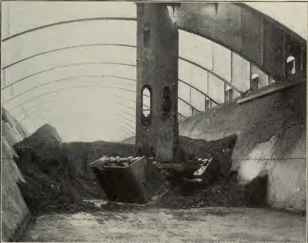
UNLOADER LEG AND BUCKET OF HULETT AUTOMATIC UNLOADER IN THE HOLD OF AN ORE VESSEL.
