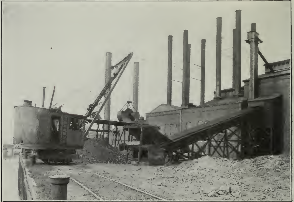
LOCOMOTIVE CRANE FOR BOILER-HOUSE COAL-HANDLING SYSTEM, PUBLIC SERVICE CORPORATION OF NEW JERSEY.
