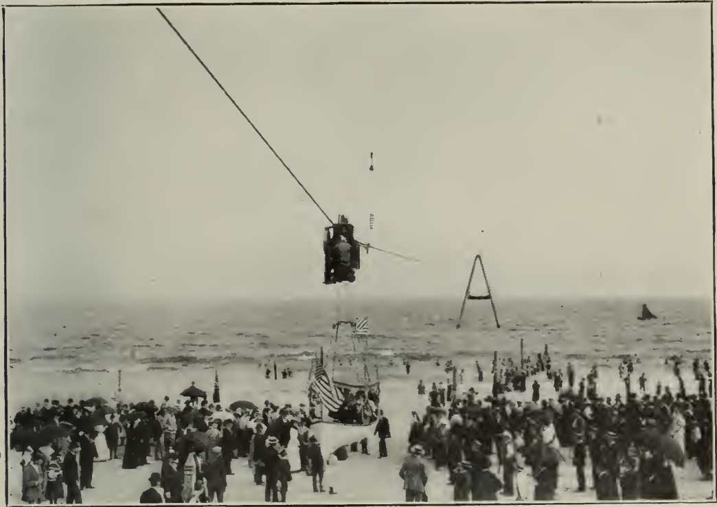
EXPERIMENTAL BALANCED CABLEWAY AT CONEY ISLAND, N. Y.
