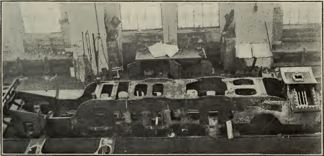
FIG. 26. PARIS-ORLÉANS LOCOMOTIVE FRAMES FOR PACIFIC TYPE.
