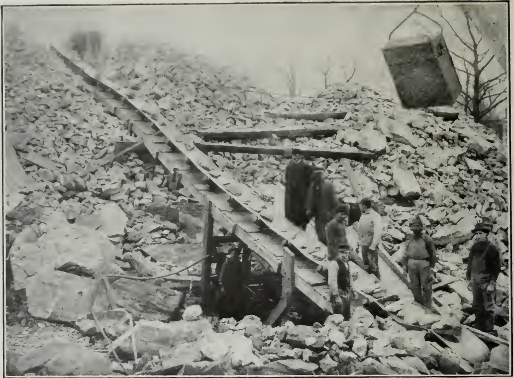
ROBINS CONVEYING BELT REMOVING EARTH AND ROCK.
