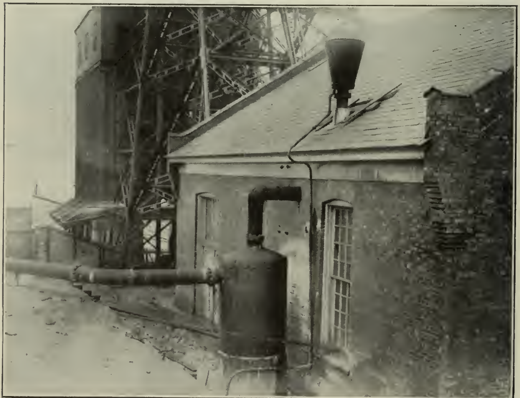
RECEIVER AT THE HOISTING-ENGINE HOUSE.
