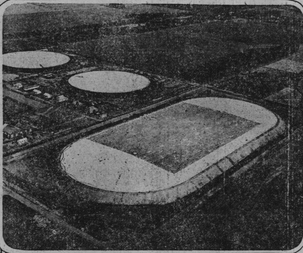
OIL, OIL, OIL —Aerial view of huge concrete reservoir near Los Angeles which holds nearly 2,000,000 barrels, while the smaller ones hold half a million each.
