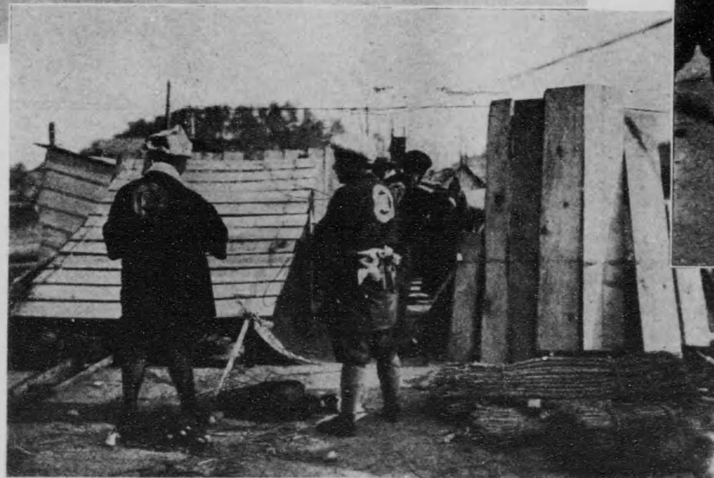
Installing electric lights in the shacks (Toyo-oka)
