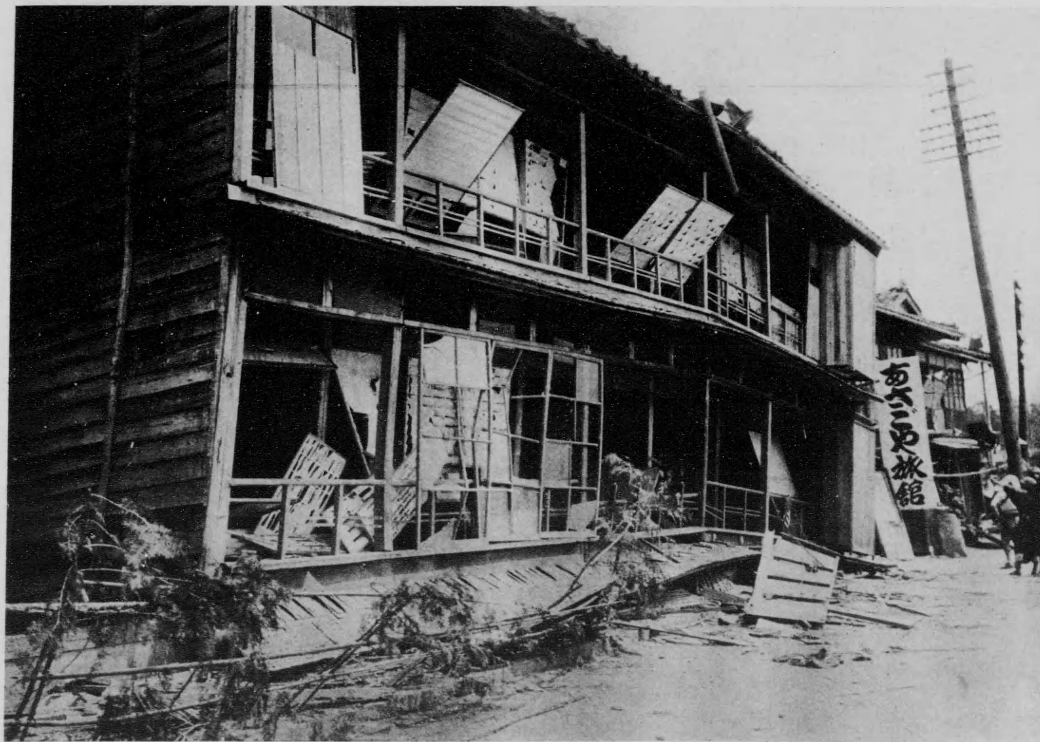
Three-storeyed hotel turned into a two-storeyed house (Kinosaki) (のもたれ潰がけ丈下の建階三) 館旅泉温の崎城
