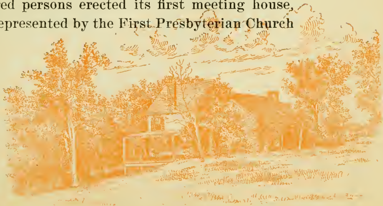
OLD STONE HOUSE AT SOUTH ORANGE.
