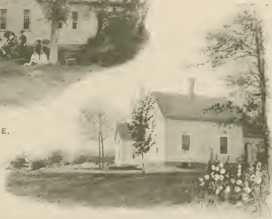
COTTAGES 1 AND 2, SOUTH OF MANSION HOUSE.
