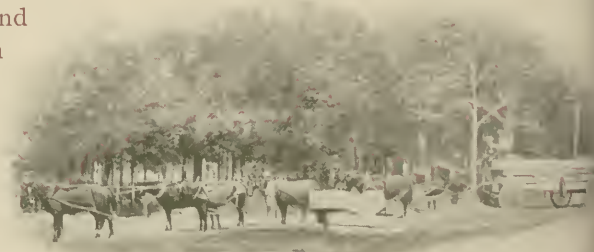
THE LARGE STEPS OF MAINE STATE BUILDING ARRIVING AT POLAND SPRING.
