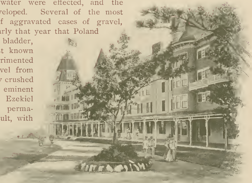
POLAND SPRING HOUSE, FROM GROVE.
