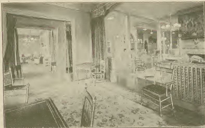
OFFICE, FROM LADIES' PARLOR AND READING ROOM.
