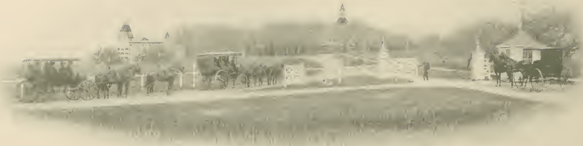
ENTRANCE TO POLAND SPRING HOUSE AND PARK, FROM MANSION HOUSE.
