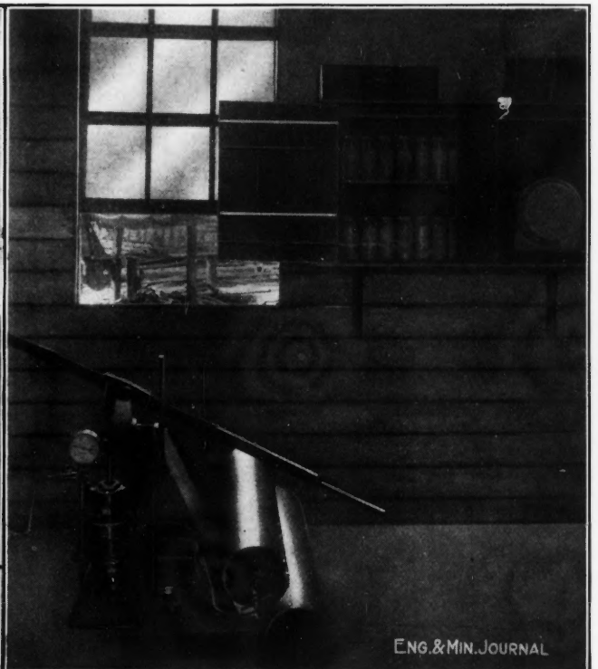
ANOTHER VIEW OF EQUIPMENT ROOM
