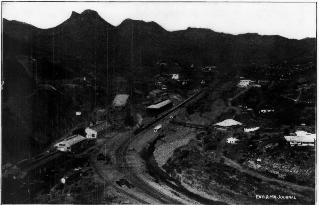
GENERAL VIEW OF MINE PLANT, SHOWING NO. 1 SHAFT Ore is shipped over Ray & Gila Valley R.R. to Kelvin, thence over the Arizona Eastern to the mill at Hayden, 16 miles distant.
