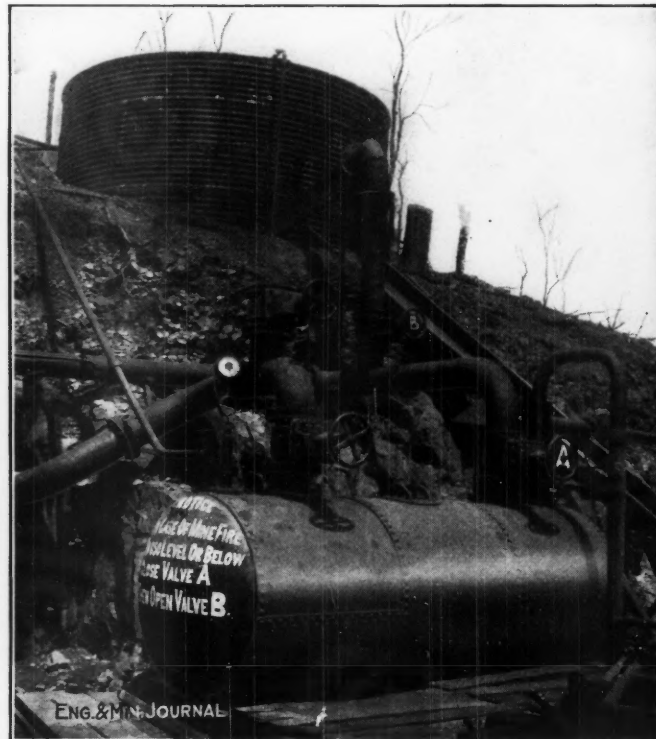
AN OUTSIDE STORAGE TANK AND CONNECTIONS
