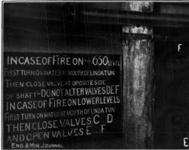
TYPICAL SET OF VALVES AND INSTRUCTIONS UNDERGROUND
