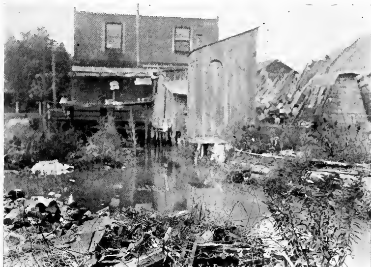
Fig. 41.—Sewage in the interior of a village block that needs a public sewer system.
