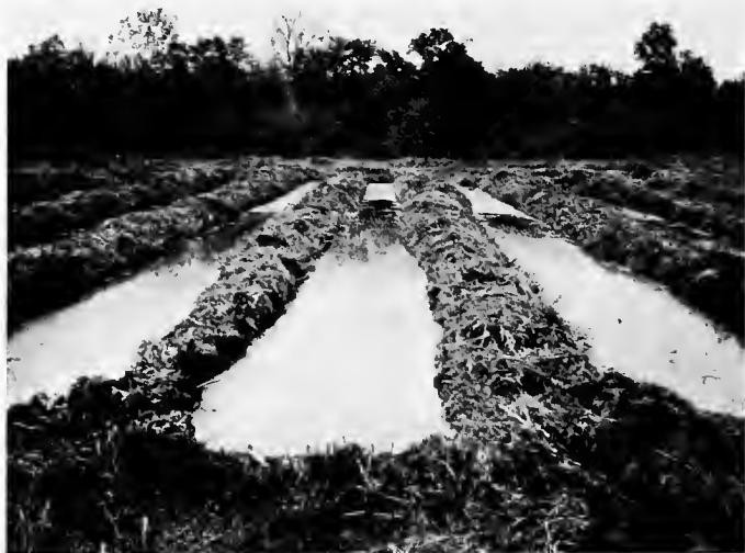
Fig. 42.—Surface disposal of sewage—a crude system.
