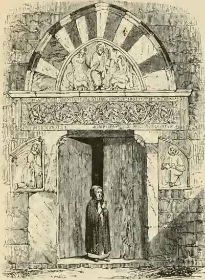
478. Doorway in Church at Maguelone. From Renouvier, Monumens de Bas Langue loc.
