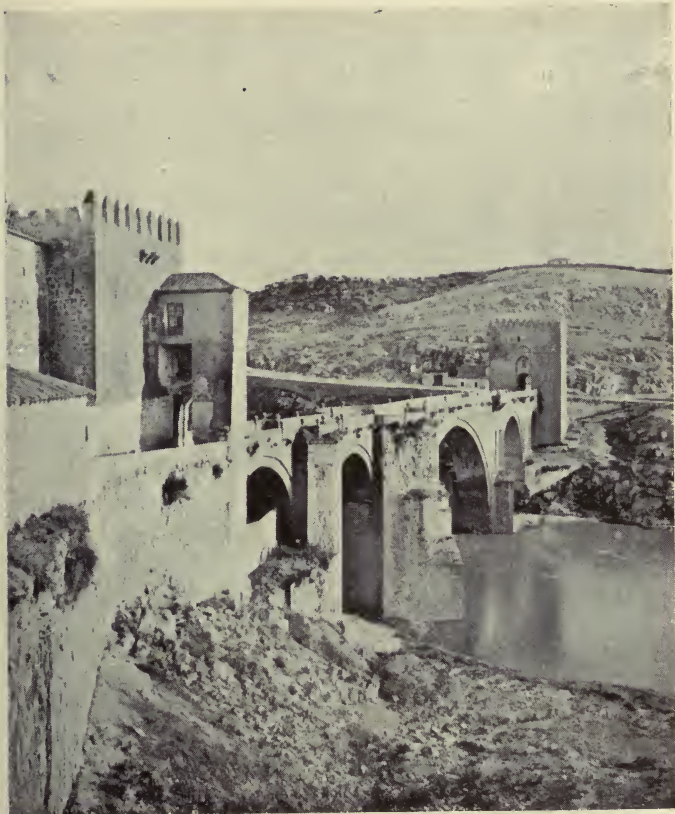
ST. MARTIN'S BRIDGE.
