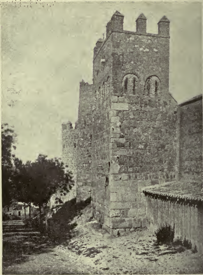
TOWER IN THE CITY WALLS OF "THE SUBURB OF SAN ISIDORO," NEAR THE NEW BRIDGE OF VISAGRA
