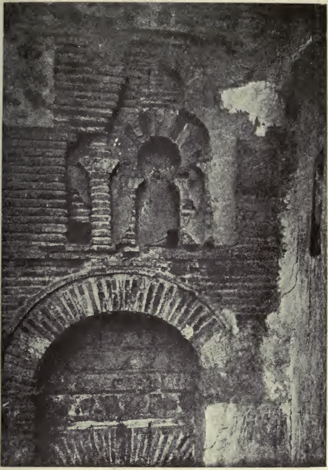
THE MOSQUE OF BIB-AL-MARDÓM, HORSE-SHOE ARCH AND REMAINS OF THE DADO OF LITTLE ARCHES AND WINDOWS IN THE NORTH-EAST FAÇADE (LEFT SIDE)
