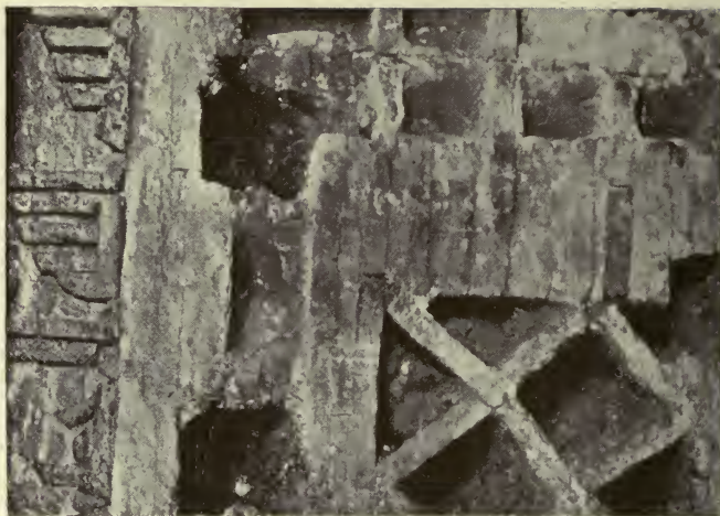
DETAIL OF THE NORTH-WEST FAÇADE OF THE MOSQUE OF BIB-AL- MARDÔM
