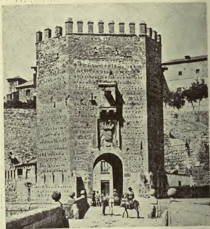
DEFENSIVE TOWER OF THE BRIDGE OF ALCANTARA. ANTERIOR FAÇADE
