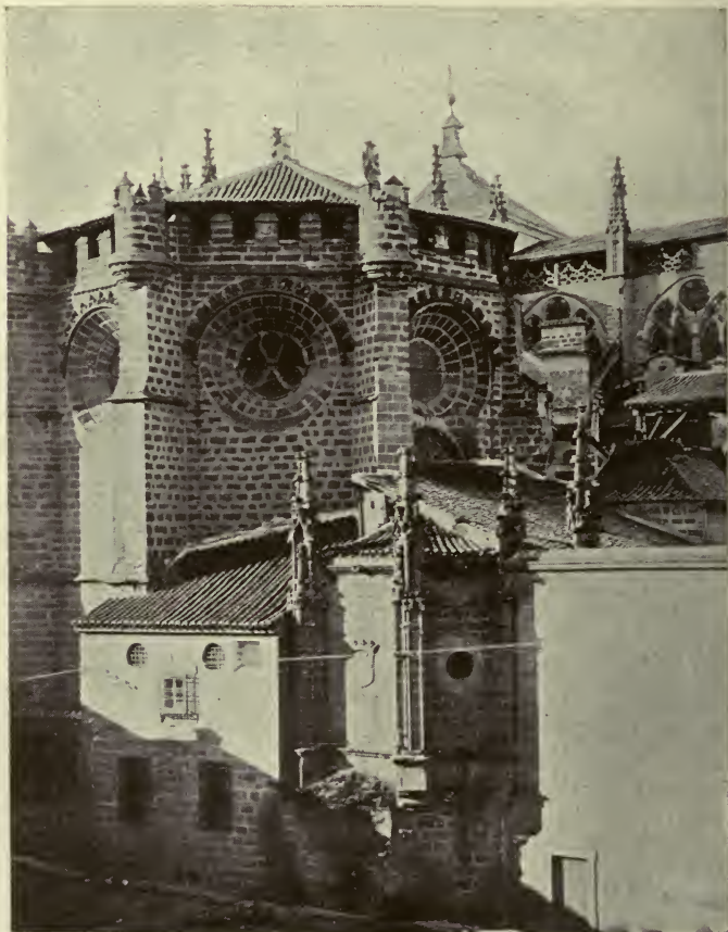
THE CATHEDRAL. DETAIL OF THE EXTERIOR
