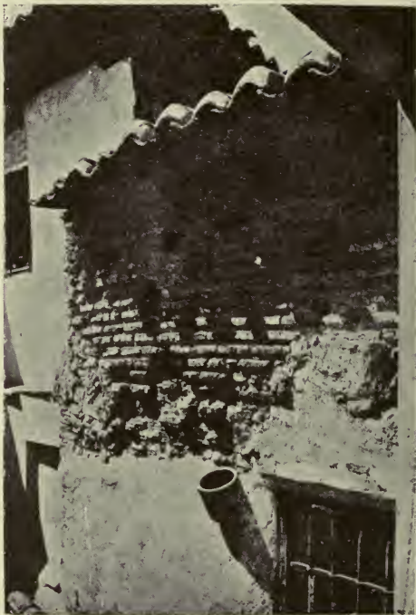
MOSQUE OF THE TORNERIAS. EXTERIOR OF THE SOUTH FAÇADE, SOUTH-WEST ANGLE
