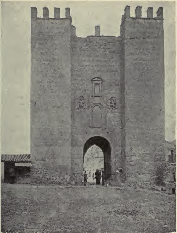
POSTERIOR FAÇADE OF THE DEFENSIVE TOWER OF THE BRIDGE OF ALCANTARA
