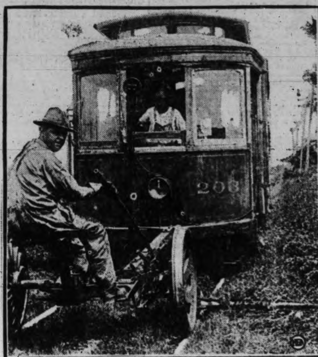
NOVEL WEED BARBER. —Scythe welders, look to your jobs. An interurban railway in Rockford, Ill., now cuts all the weeds along its right of way with a mower hooked on behind a trolley car, accomplishing the work of hundreds of men at a fraction of the cost.
