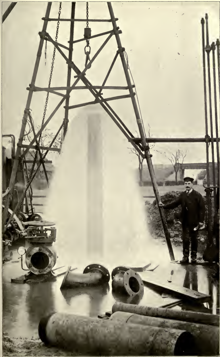
A TYPICAL ARTESIAN BORING.
