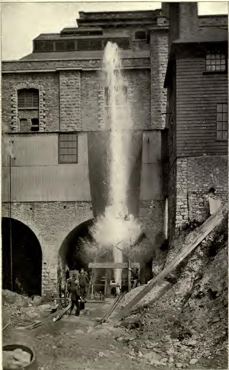
EXPLODING A CARTRIDGE IN A DEEP BORING TO INCREASE THE YIELD OF WATER.
