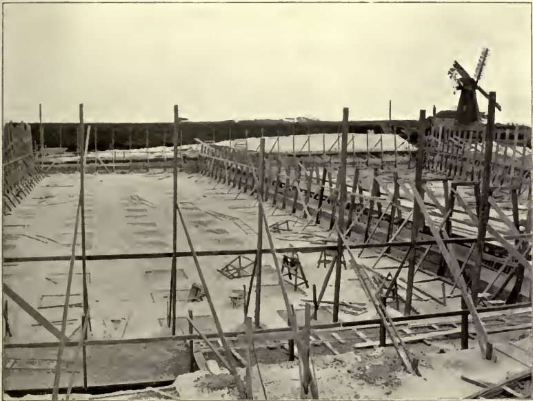
A COVERED SERVICE RESERVOIR, 5,000,000 GALLONS CAPACITY, IN COURSE OF CONSTRUCTION.
