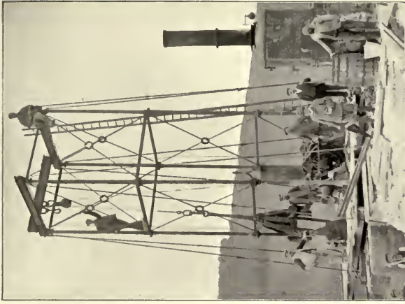
THE AUTHOR AND MEN BORING WITH A 60-INCH CHISEL.
