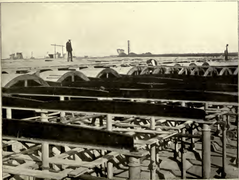
THE IRON COLUMNS AND GIRDERS THAT SUPPORT THE ROOF, WITH THE CENTERING TO FORM THE ARCHES.
