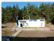
Novoverbivka Railway Crossing Loop Building (2018) 01.jpg
