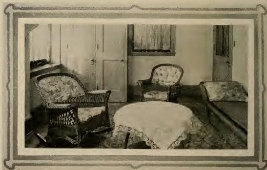
Ladies Rest Room on second floor of the "Perfection" office building
