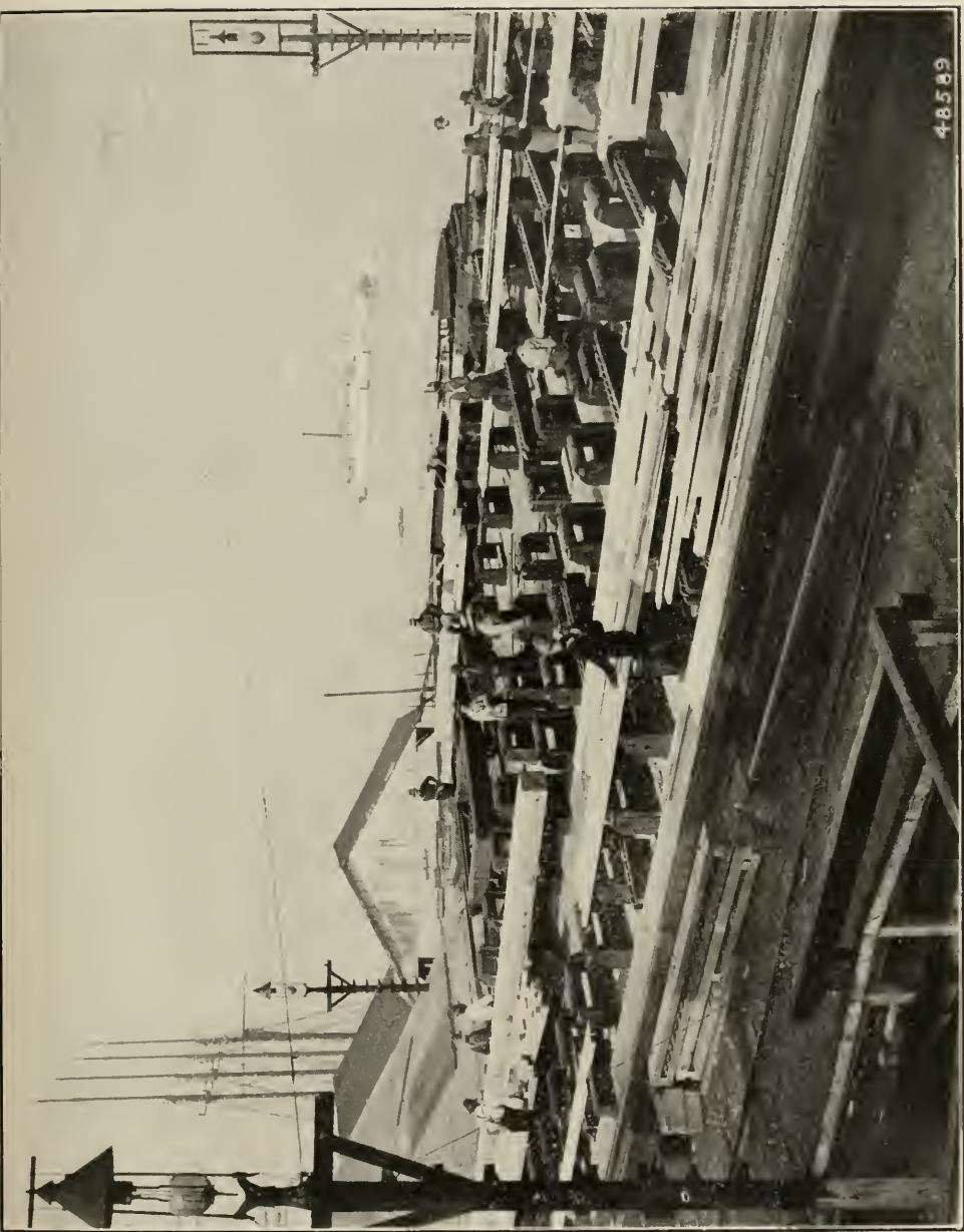
A LUMBER WHARF SCENE AT TACOMA, WASH., WITH THE ROLLERS ON WHICH DOUGLAS FIR PLANKING AND HEAVIER TIMBERS MAY BE READILY HANDLED. IN THE DISTANCE A STERN WHEEL STEAMER OF THE TYPE COMMON ON PUGET SOUND AND THE RIVERS WHICH EMPTY INTO IT.
