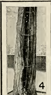
No. 4.—A long cavity with nails and cement reinforcing rods in place ready for filling. This cavity should have been bolted.
