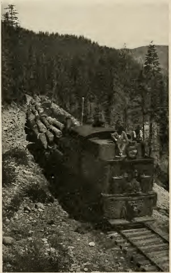
DOWN GRADE WITH A HEAVY LOAD OF LUMBER.
