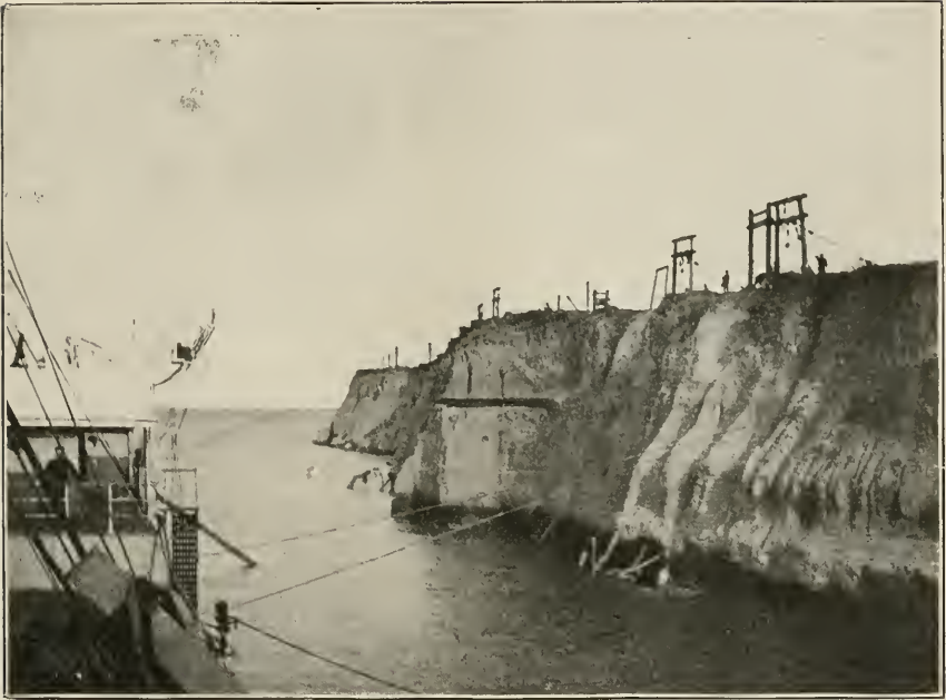
LOADING QUEBRACHO FROM A HIGH RIVER BANK TO AN OCEAN-GOING STEAMER. On the Paraná River, near Rosario, anchorage is found for steamers of considerable draft, but special apparatus is employed to get the logs on board. They are first lowered to the stream by wire rigging and then hoisted to the deck.
