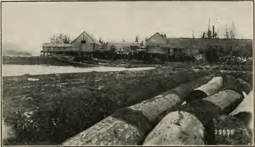
SITKA SPRUCE LOGS IN THE SAWMILL, BOX FACTORY AND BOAT BUILDING PLANT AT PORT GRAVINA ISLAND, ALASKA.
