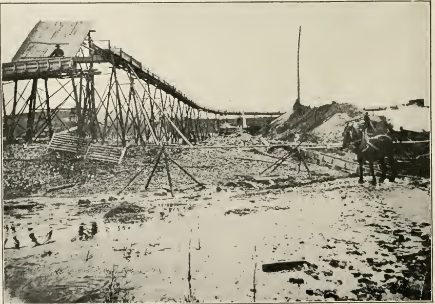
TYPICAL FLUME AND SLUICE BOXES USED IN PLACER MINING FOR GOLD IN THE FAIRBANKS DISTRICT. MUCH LUMBER AND MANY POLES ARE REQUIRED FOR THESE PURPOSES.
