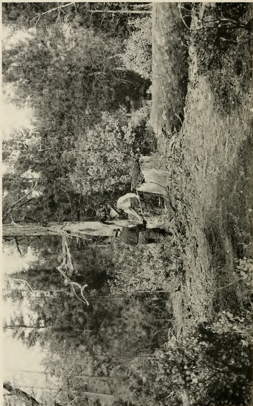
A SNAG FELLED BY POWDER, SHOWING METHOD OF QUICK WORK IN CLEARING A WAY THROUGH THICK GROWTH FOR A FIRE LINE.
