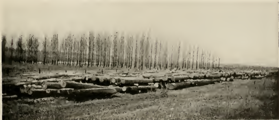
THE RIVER BANK IS LINED WITH LOGS.
