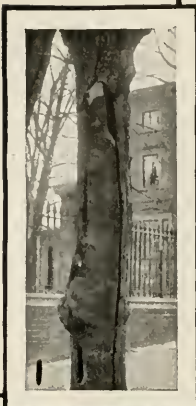
No. 1.—Cement filling shattered by cold weather and swaying of the tree.
