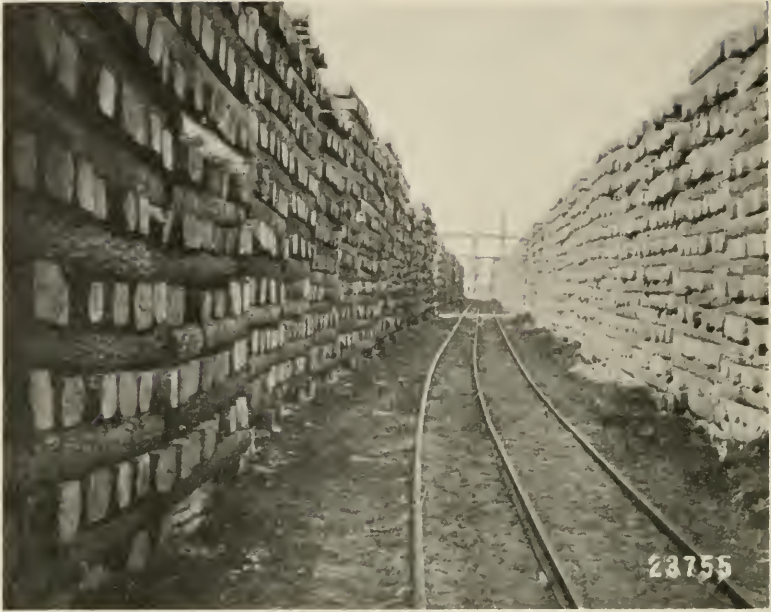
UNTREATED TIES PILED IN YARD AND TRAM TRACKS, ESCANABA, DELTA COUNTY, MICHIGAN. There has never been a successful substitute for the wooden tie and engineers are willing to admit there never can be. When treated with preservatives a large measure of permanence is added to their other good qualities.
