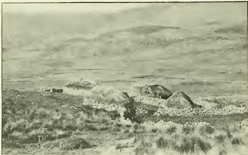
A GROUP OF NATIVE HOUSES AT THE UPPER LIMIT OF CULTIVATION, PASS OF LA RAYA, SOUTHERN PERU.
