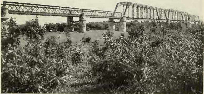
VIADUCT CONSTRUCTION IN SOUTH AMERICA
