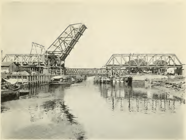
BRIDGE CONSTRUCTION IN SOUTH AMERICA
