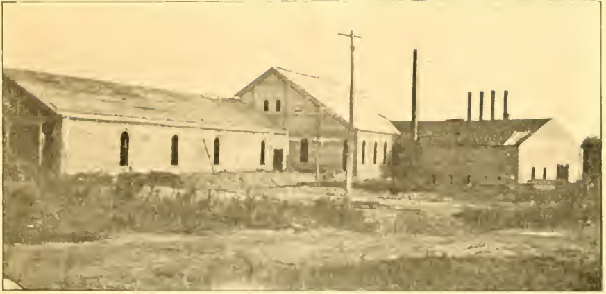
NORWOOD POWER PLANT.
