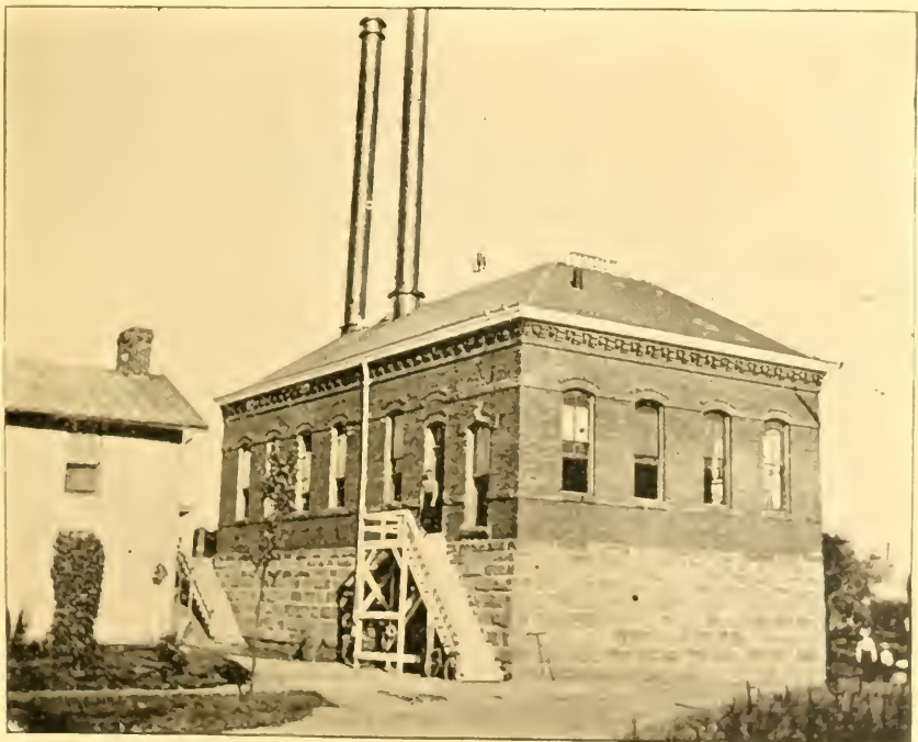
PUMPING STATION CITY WATER WORKS.
