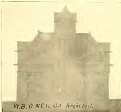
HOSE HOUSE NO 2.
