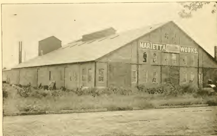
MARIETTA BOILER WORKS.
