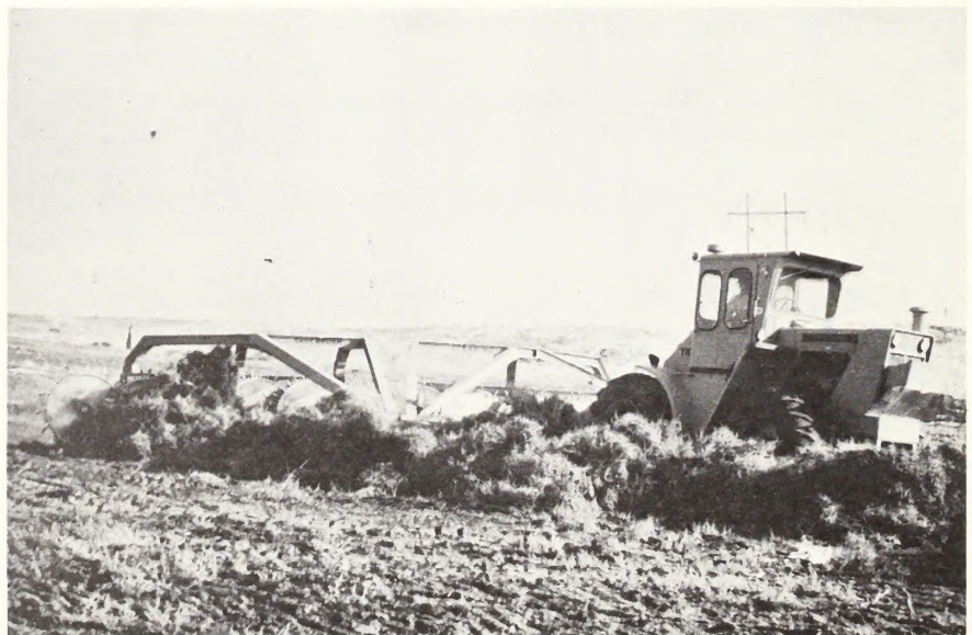
FIGURE 1-2. A brush rake being used to windrow brush for burning in preparing the land for plowing.
