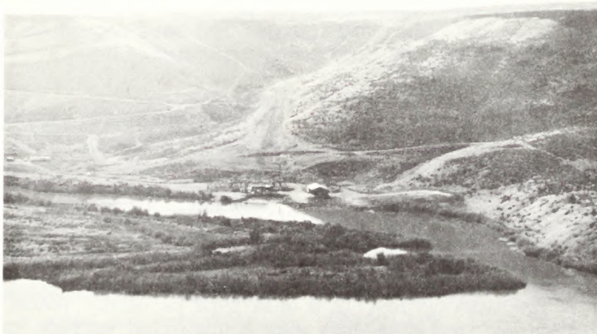
FIGURE 1-5. Aerial panorama of pump station located on a side channel of the Snake River. A buried penstock ascends the hill behind the station to deliver irrigation water to the bench high above the river.
