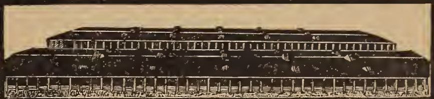
Storage Sheds of Chippewa Beet Sugar Co. 100,000 sq. ft. of Black Diamond Roofing.
