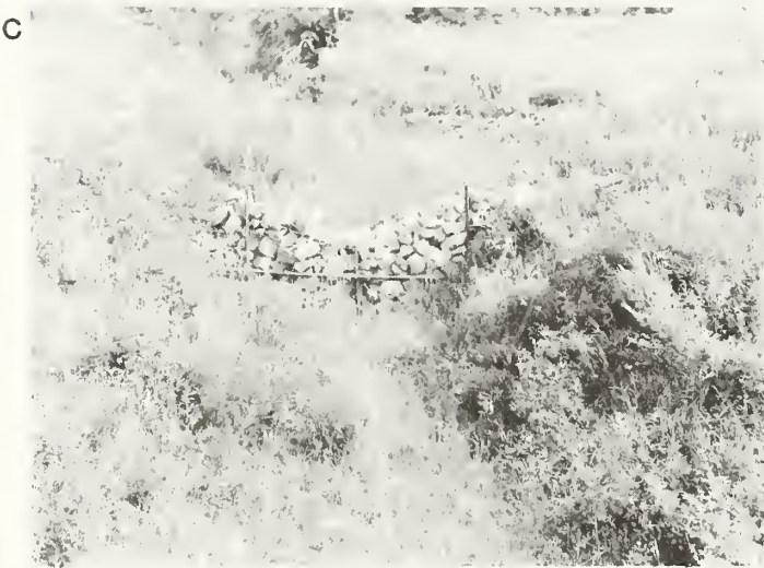
Figure 4.—An upstream view of a rock check dam constructed in an upper watershed channel on Alkali Creek in western Colorado: (a) immediately after construction in 1963, (b) in 1964, and (c) 12 years later in 1975. Notice the establishment of grass on channel banks and bottoms but the absence of riparian plants.
