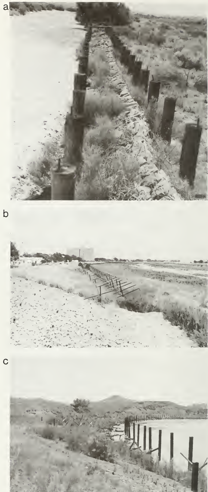
Figure 12. — Commonly used bank armoring and protection devices: (a) revetment posts and gabion near Moab, Utah; (b) jacks and bank armor at Dodge City, Kansas; and (c) jack field behind revetment posts on the Powder River, Wyoming.
