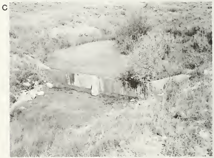
Figure 5.—The appearance of the site occupied by a larger gully control structure at the mouth of Alkali Creek in western Colorado: (a) immediately after treatment in 1963, (b) in 1964, and (c) 12 years later in 1975.
