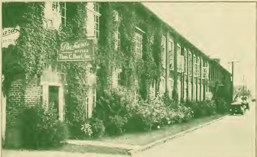
Hundreds of bare brick walls in the South should be screened
