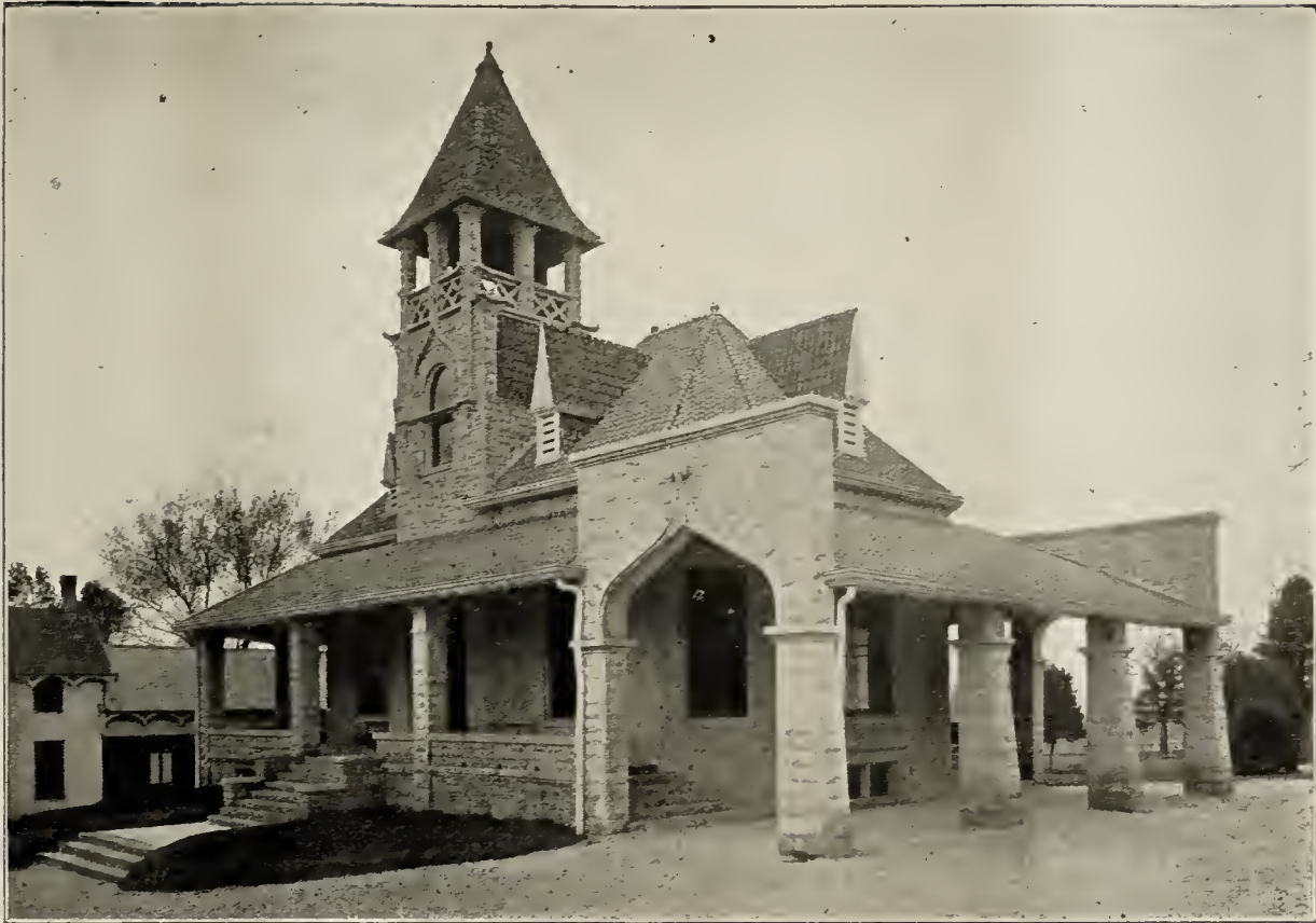
ADMINISTRATION BUILDING, OAK HILL CEMETERY, EVANSVILLE, IND.
