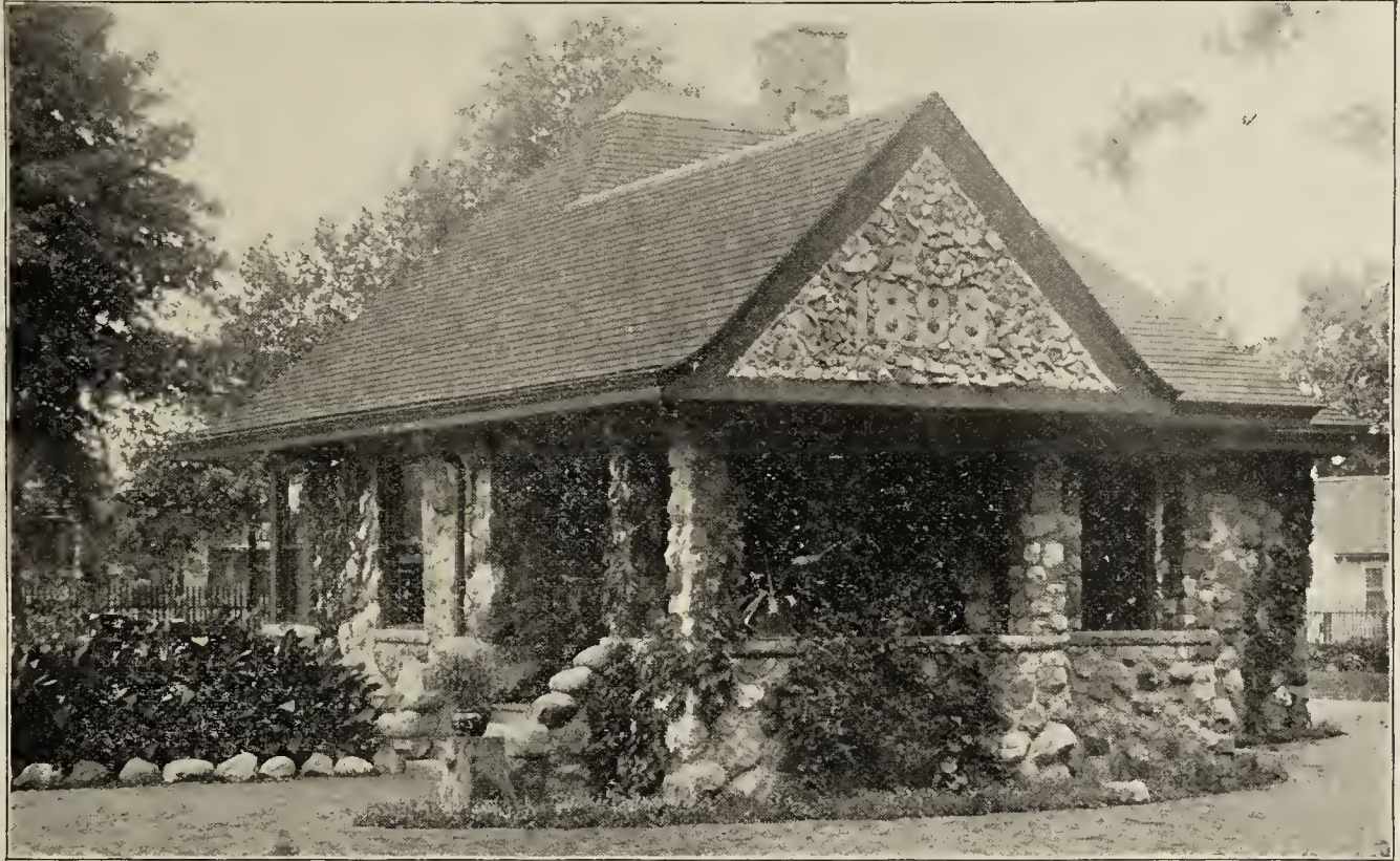
ENTRANCE AND OFFICE BUILDING, BLOOMINGTON CEMETERY, BLOOMINGTON, ILL.
