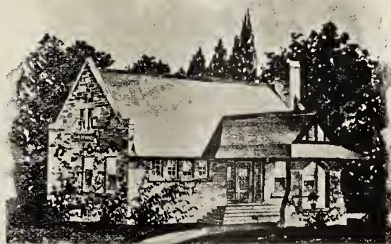
OFFICE BUILDING, LAKE VIEW CEMETERY, CLEVELAND, O.
