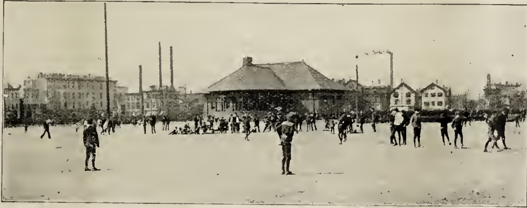
GRAVEL PLAYGROUND AND FIELD HOUSE.
