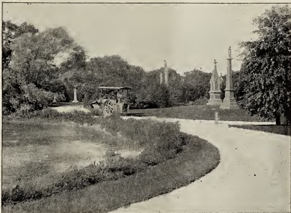
ROAD ROLLER AT WORK IN SPRING GROVE CEMETERY, CINCINNATI, O.
