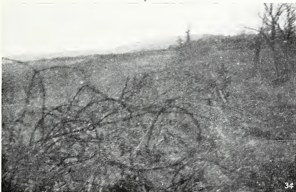
34. Another type of wire entanglement. This was placed by being stretched out like an accordion
