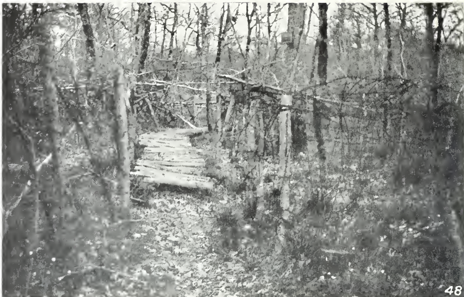
48. Close up of wire showing the beginning of the zig-zag path through the entanglement. This was their main line of defense and, of course, the outposts had to have a quick way of getting through when pressed. This path is raked by the machine-gun position shown in No. 49
