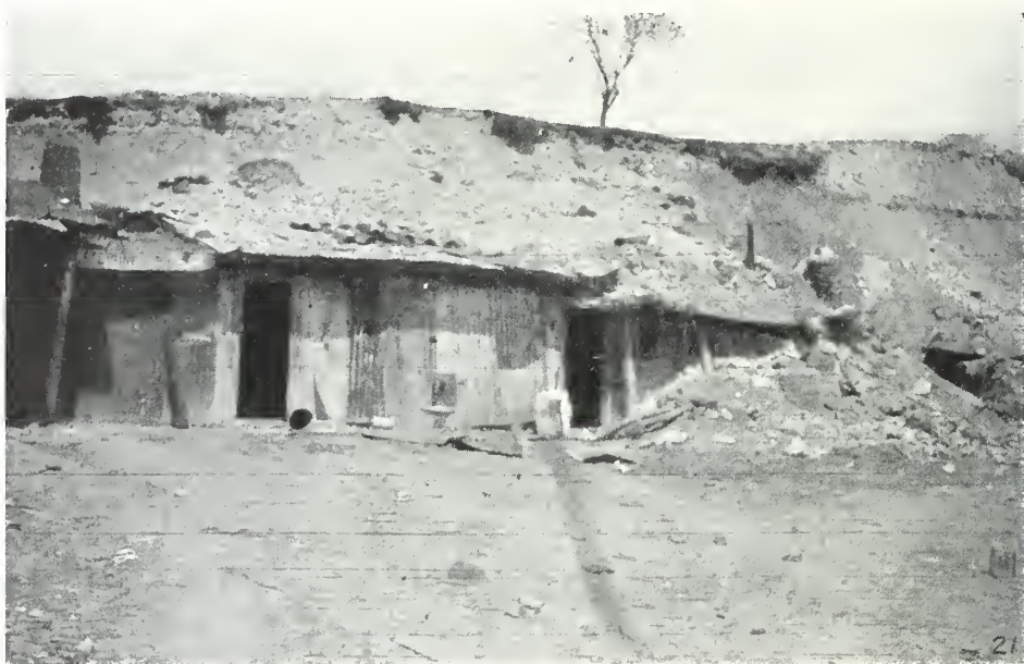
21. One of the company kitchens was located here by the roadside at Bordeaux
