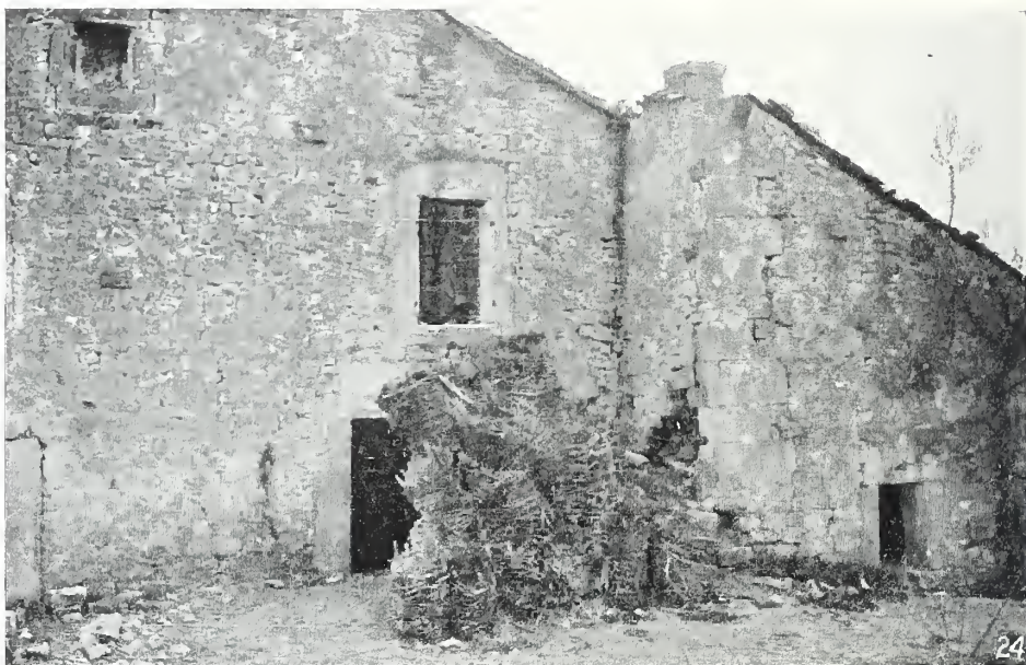
24. Within the door at the center just behind the barricade was the 323d Infantry dressing station near Haudiomont. This is just across the road from No. 23
