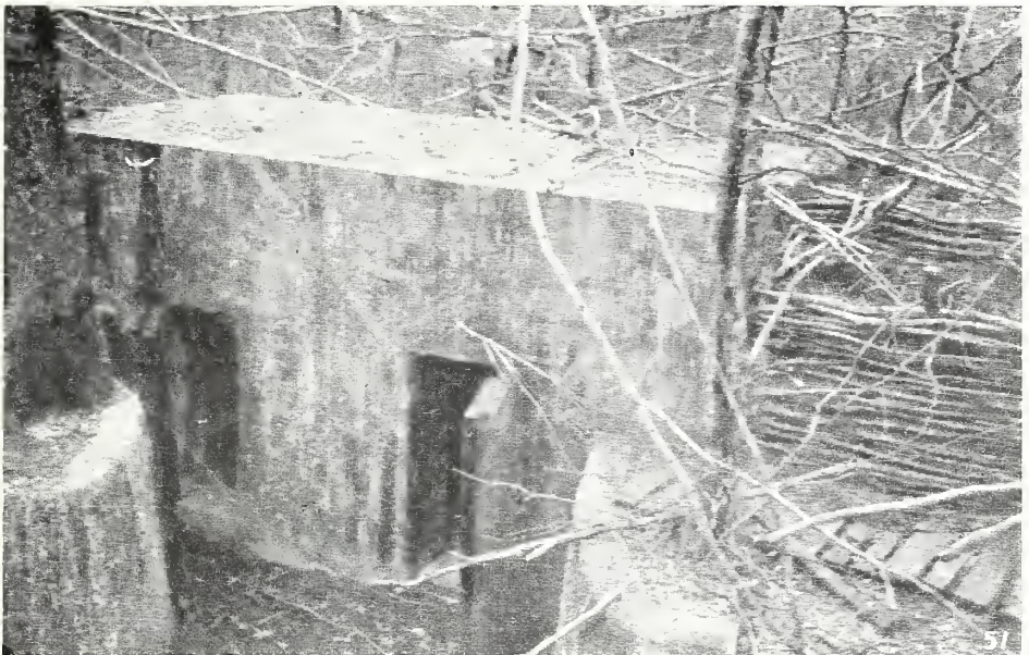
51. No. 49 machine-gun nest seen from behind. Note the thickness of the walls and roof
