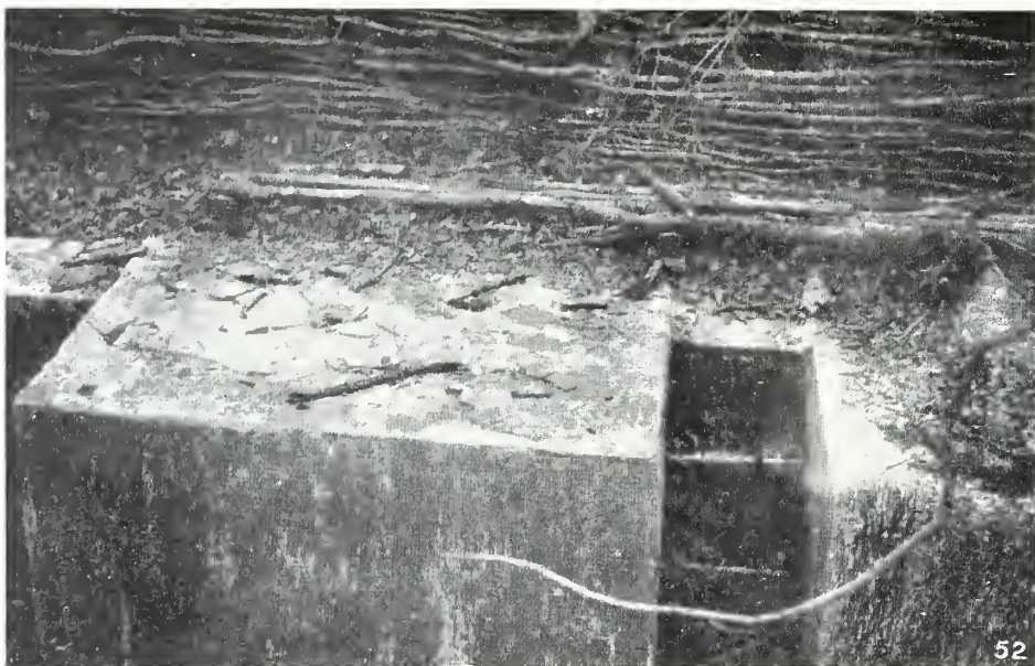
52. Concrete top of dugout in trench near machine-gun nest seen in No. 49
