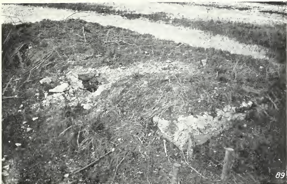
89. Two direct hits on the dugout shown in No. 88. It was a three-inch shell that did this. One went right through the roof
