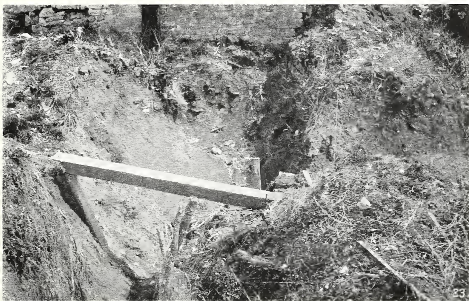
23. This trench was about ten feet deep. Across the beam (6x6 inches) shown here, many of the wounded were brought out to ambulances on the road near Haudiomont during the night of November 9th. The road is just outside the picture at the right. The third battalion dressing station was in a dugout in the front-line trenches at the bottom of a steep hill at the left. Can the tortuous wire entanglements and maze of communicating trenches of that hill ever be forgotten?
