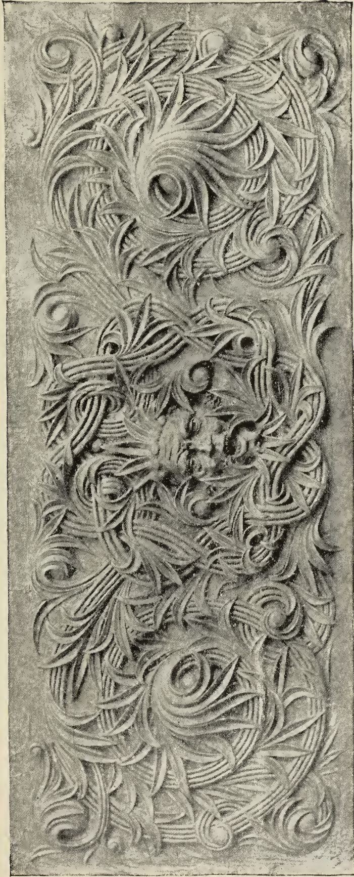
206.—PANEL IN WAREHOUSE, JERSEY CITY, N. J. PERTH AMBOY TERRA-COTTA COMPANY.
