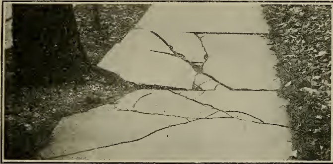
FIG. 11. Tree breaking a concrete walk.
