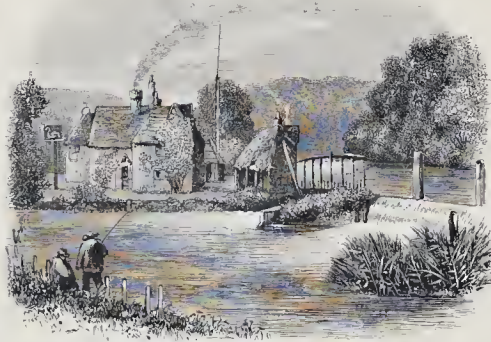
No. 15.—Pangbourne Weir.
