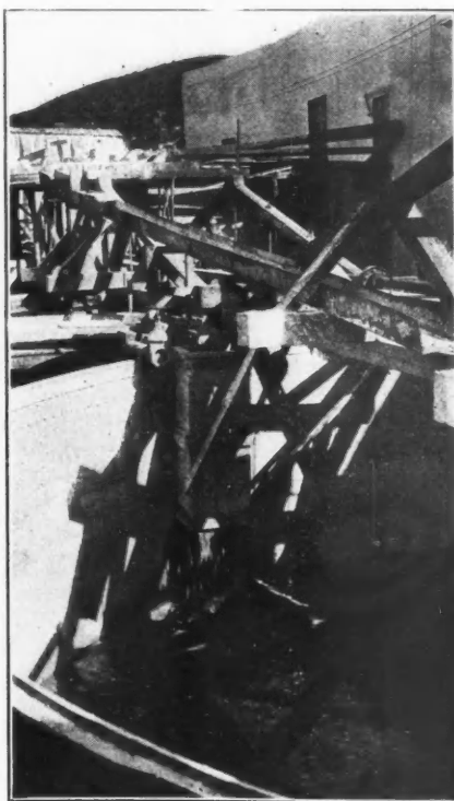
SLIME TANK, CHARGING BOX; LAUNDRER USED FOR PUMP CIRCULATION; FLORES MILL
