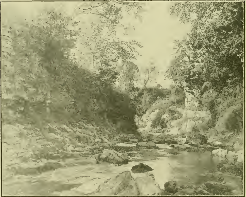
FIG. 1. Looking down the Gorge towards the site of the old Woolen Mill, just above the Waterfall.
