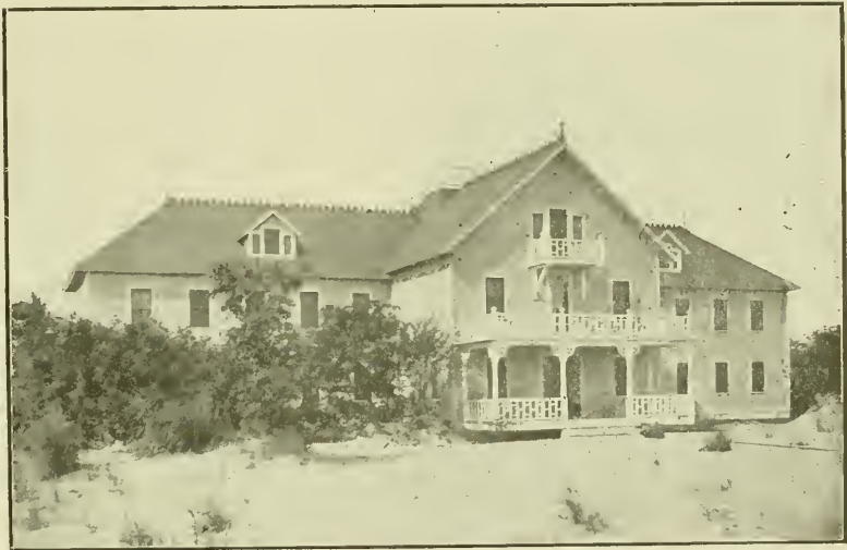
THE LAKE LABORATORY BUILDING. (Photo by Herbert Osborn.)
