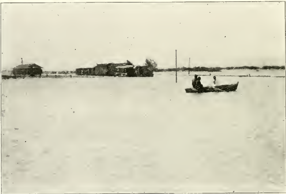
THE STATION AT MEXICALI, MEXICO, AND R. R. GRADING CAMP ON JUNE 4.
