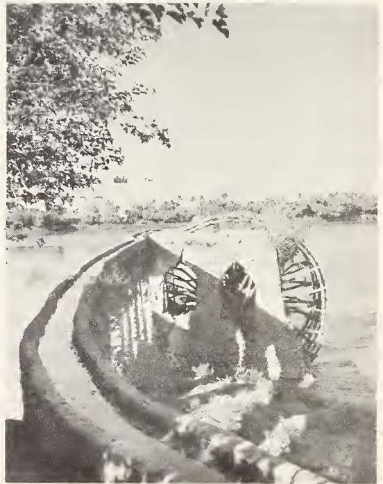
Figure 5.--Euphrates waterwheels of ancient design lifting water for irrigation. Iraqi Government.
