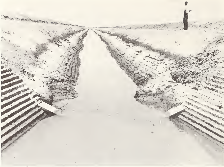
Figure 6.--Diyala irrigation canal. Note deposit of salt on banks. Iraqi Government.
