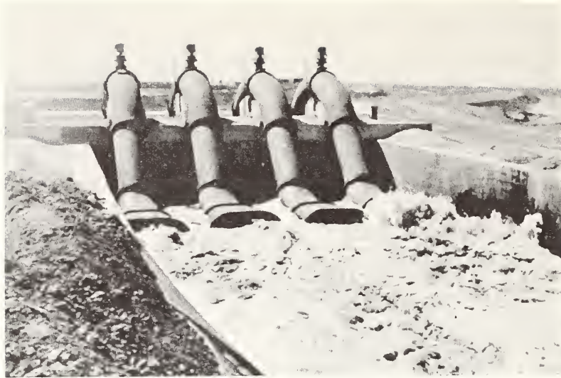
Figure 9.--Drainage regulators such as this one near Abu Ghraib drain off water carrying salt from the land. Iraqi Government.
