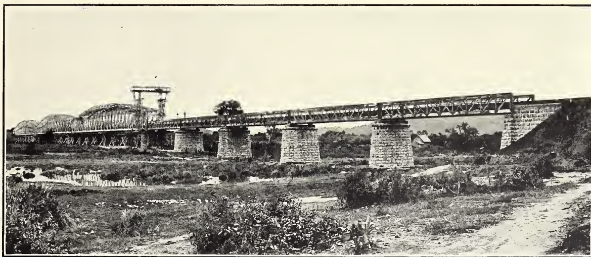
BRIDGE OVER THE IGUASSÚ RIVER.
