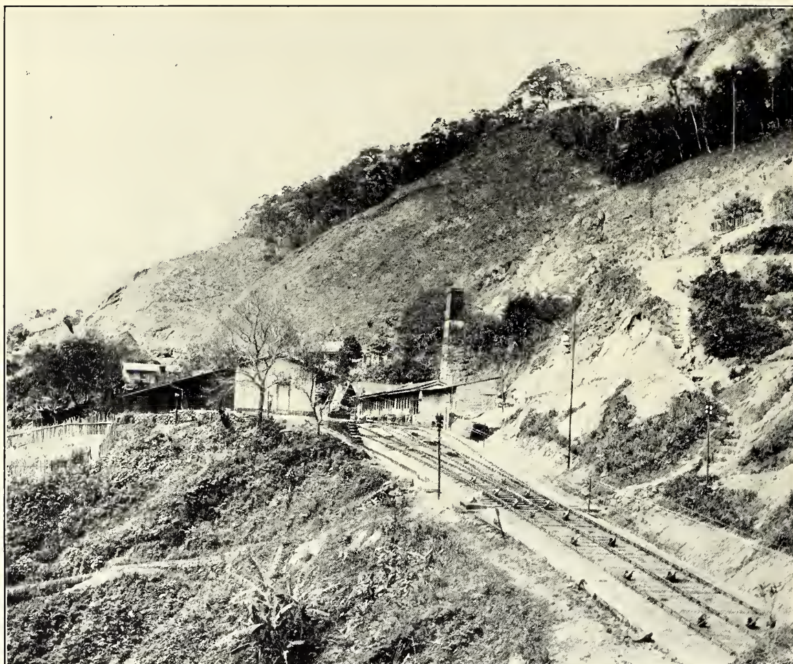
CABLE ROAD BETWEEN SÃO PAULO AND SANTOS.
