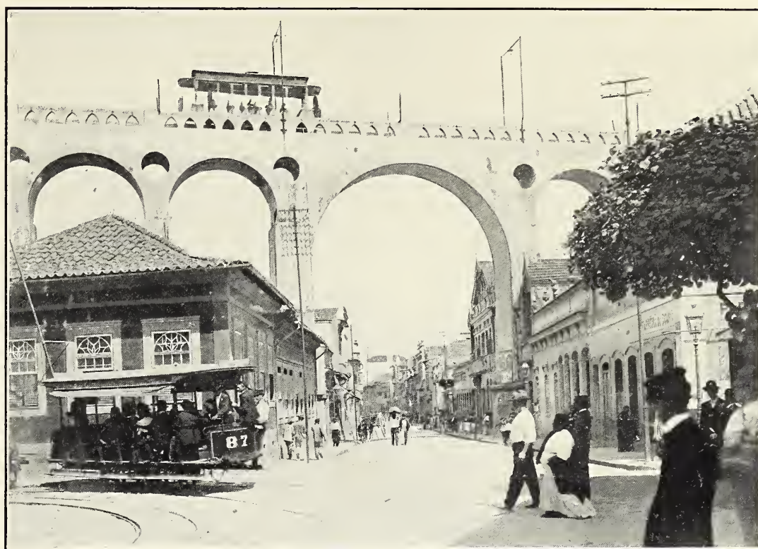
OLD CARIOCA AQUEDUCT SEEN FROM BELOW
