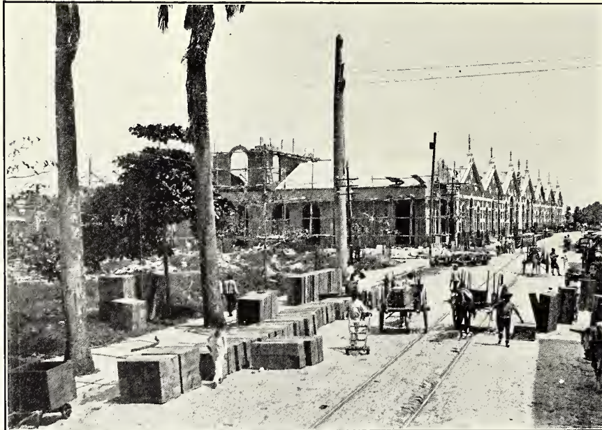
CUSTOM HOUSE, PARÁ
