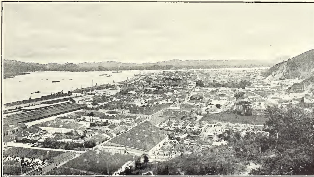
TERMINUS OF THE SÃO PAULO RAILWAY AT SANTOS, SHOWING THE DOCKS.
