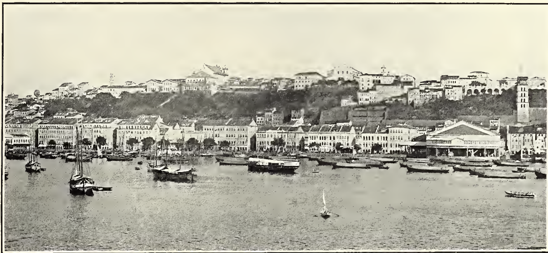
GENERAL VIEW OF BAHIA.
