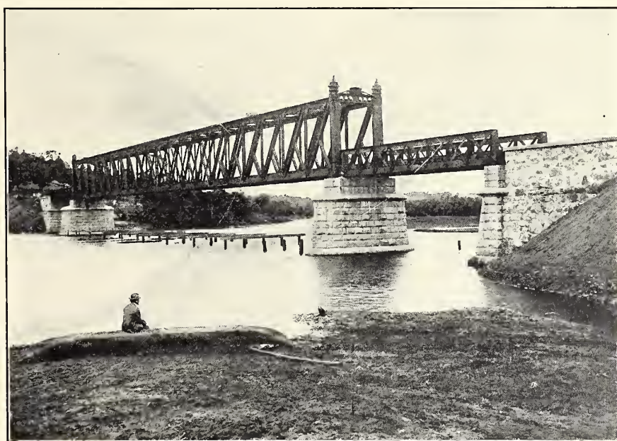
RAILROAD BRIDGE OF CASTRO, STATE OF PARANÁ.
