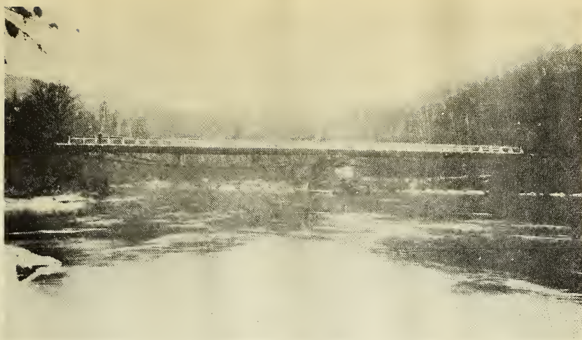
Figure 1. - The completed temporary combination timber and cable-truss bridge across the Winooski River near Middlesex, Vt.
