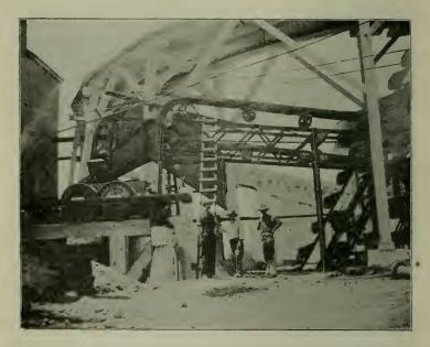
Wesselton Washing Plant, showing Trestle, Belt Conveyor, Toothed Rolls and Elevator for crushed material.
