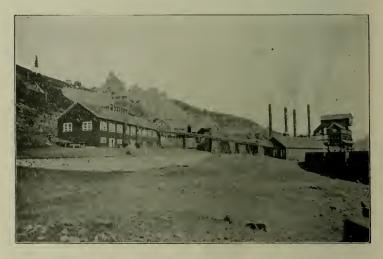
Shaft House Engine House. Aerial Tramway. Air Compressors. Black Bear Tunnel. Surtace Plant Le Roi.
