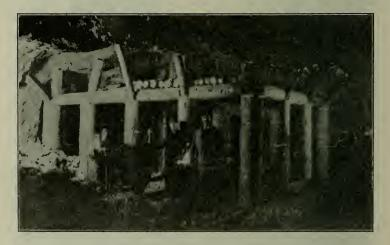
FIG. X.—The Beginning of a Stope. (Photo taken in Old Ironsides Mine)
