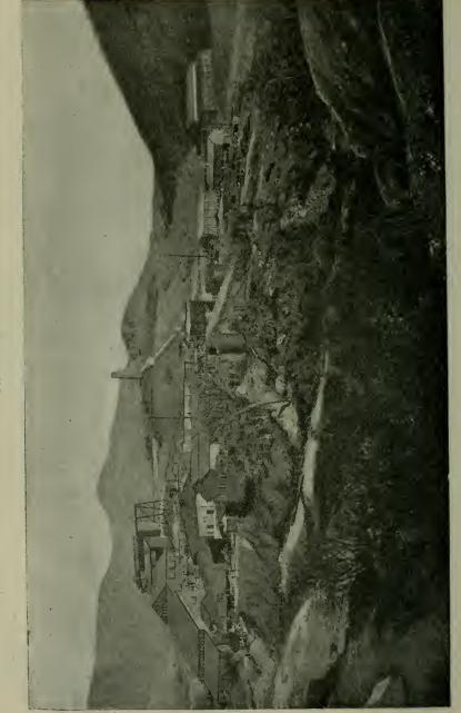
General view of Concentrating and Smelting Plant of the Moctezunia Copper Co., Nacosari, Sonora, Mexico. All the power is furnished by Loomis Gas Plant with Gas Engines and Electrical Distribution.
