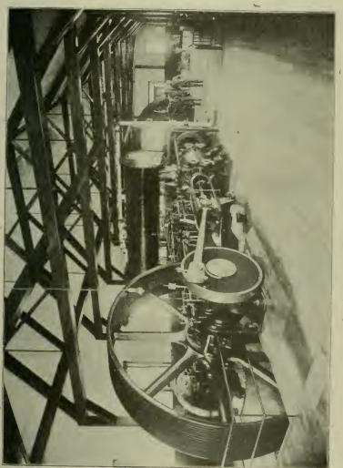
*Boiler Plant.*—This plant consists of nine horizontal, return tubular, steel shell, high pressure boilers, set in three batteries of three boilers each; and two Heine Safety Water Tube boilers set in one battery.
