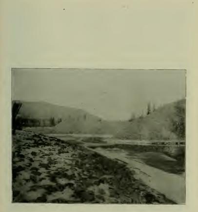
Tailings stacked up by Stacker, end of Stacker showing.
