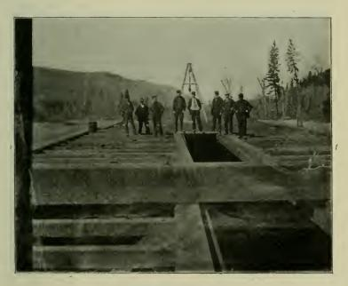
Hull of Dredge under construction.
