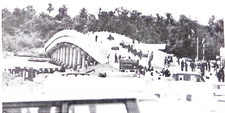
Mbo Bridge during the inspection visit by Mr President
