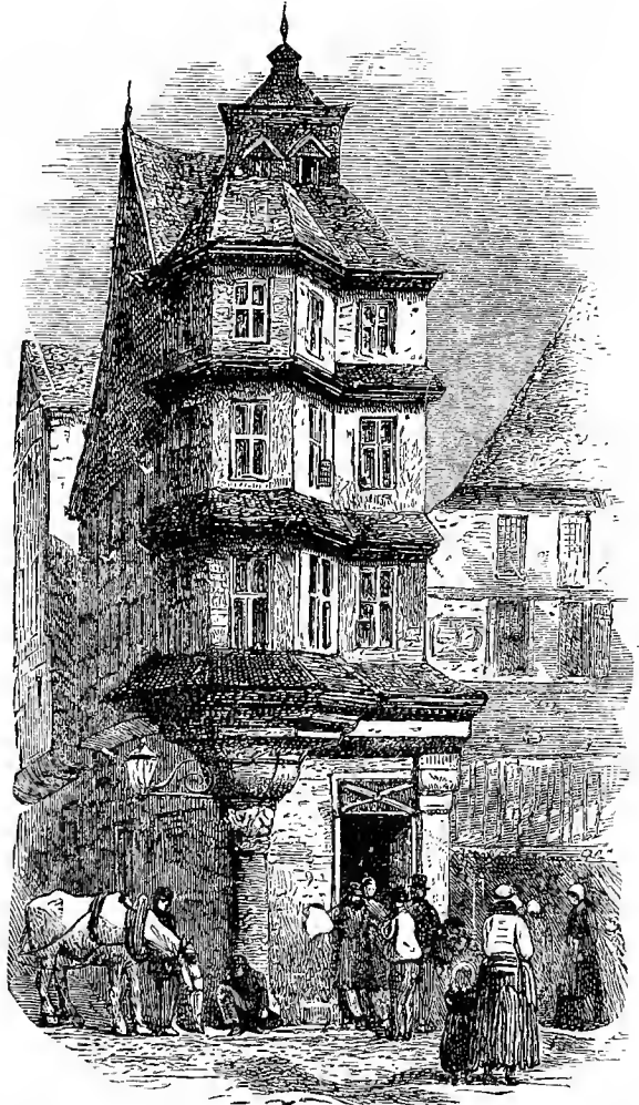
FRANKFORT: LUTHER'S HOUSE.
