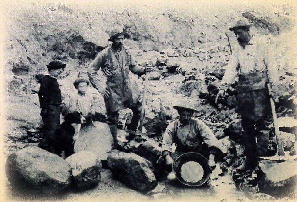
PLACER MINING FOR GOLD NEAR THE ROGUE RIVER, C. 1889.
