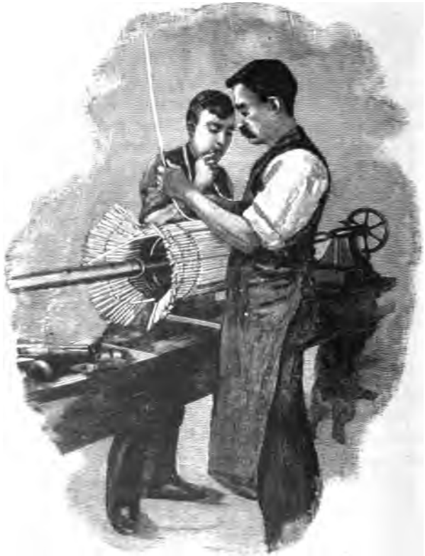
FIG. 399.—WINDING AN ARMATURE.
