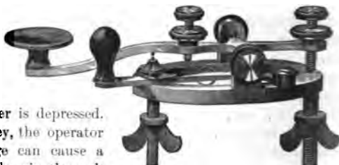
FIG. 386.—MORSE TELEGRAPH KEY.
