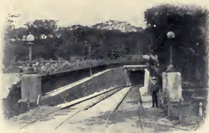
ENTRANCE TO SUBWAY, PUBLIC GARDEN
