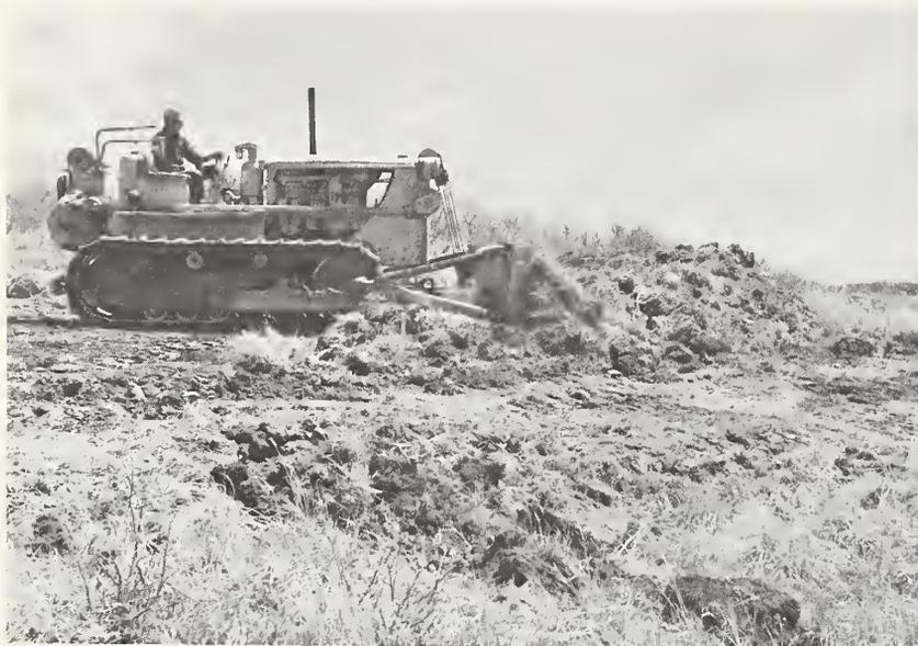
Figure 35.—Topsoil is removed from the construction area and saved, to be spread later on the finished waterway.
