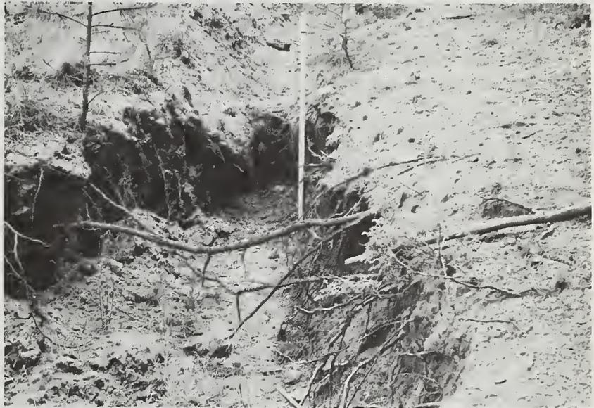
Figure 9.—The bank of Main gully, Alkali Creek watershed, 12 years after installation of check dams. Stabilization of the gully bottom made possible the invasion of dense vegetation that now is creeping up the bank. The man stands at the toe of the bank.
