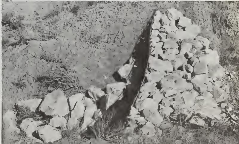
tom and side slopes to a depth that insures their stability in saturated soil. If it is impractical to drive posts to sufficient depths, the stability of the posts should be enhanced by guys. These guys should be anchored to other posts that will be covered and thus held in place by the rock fill.
