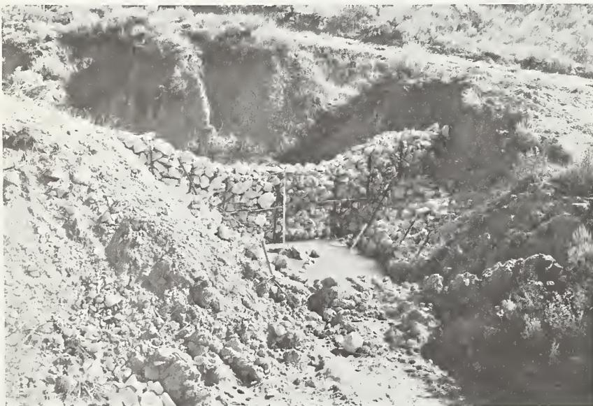
Figure 17.—Upstream view of a double-fence dam. Note the bank protection work. The apron is covered by water. Length of rod is 1.7 m.
