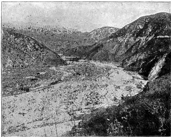
Fig. 57. Santa Ana canal on mountain side.
