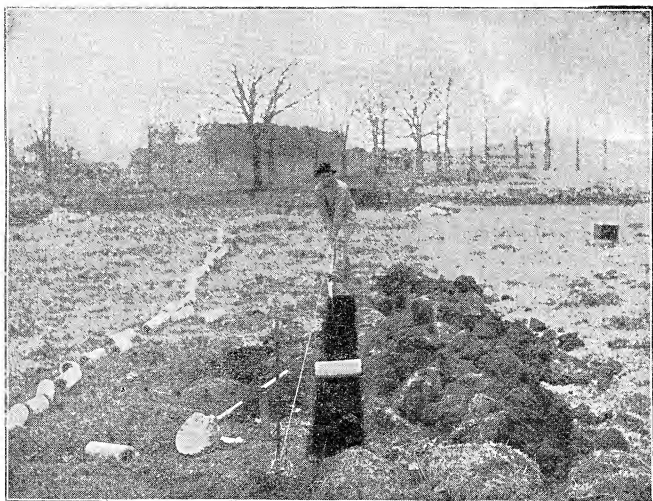
Fig. 159. Commencing a ditch.
