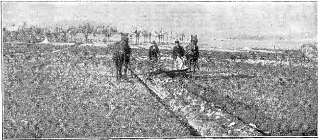
Fig. 163. The start and finish of tile draining.
