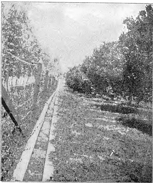
Fig. 107. Head ditch or cement flume for orange orchard, Redlands, California.
